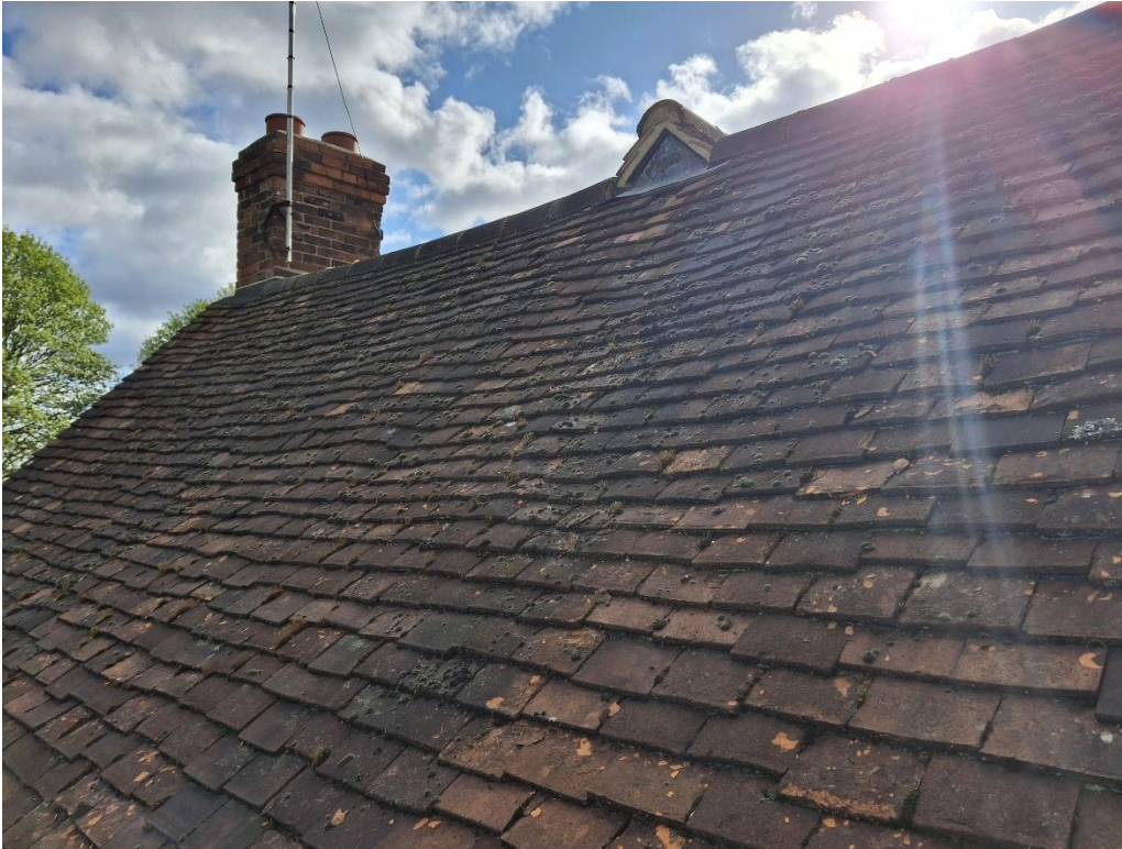
Figure 4: The northwest roof of B2, as seen from scaffolding
