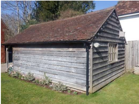
Photograph 1. Detached garage to be demolished, viewed from southeast.
