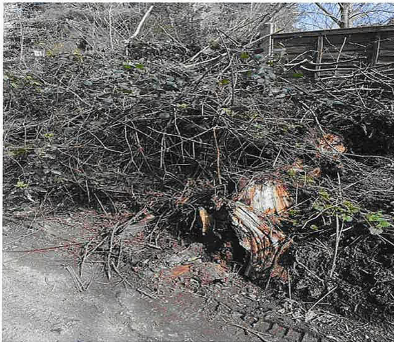
Figure 4 The damaged verge
