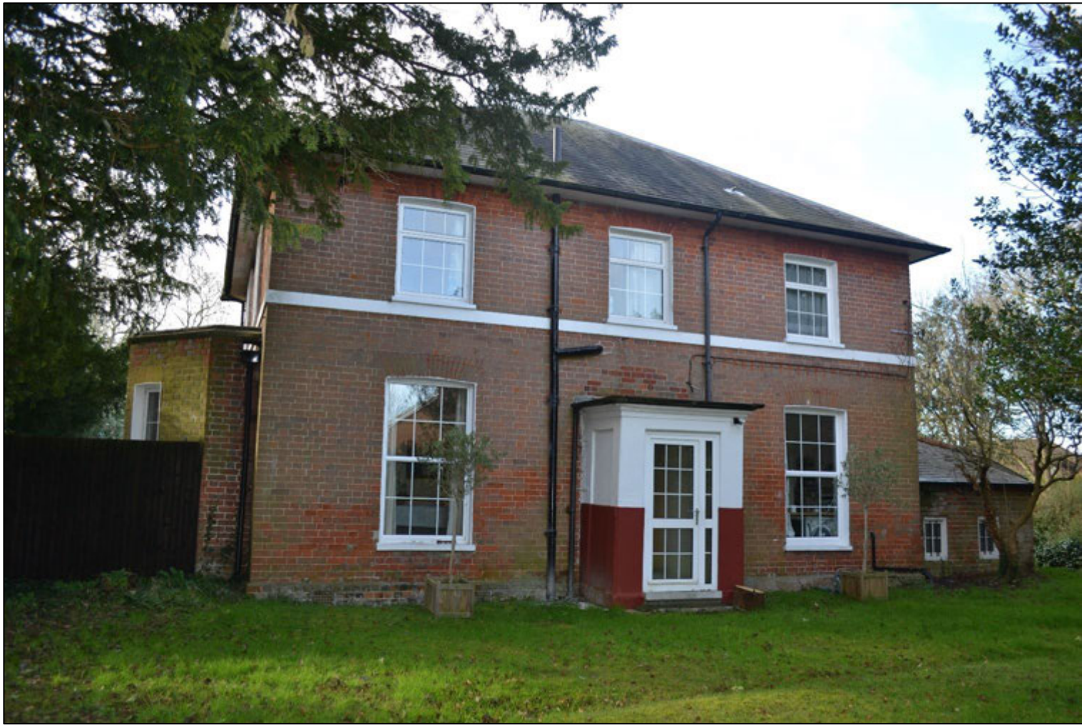
Figure 14: North (front) elevation of Sussex Lodge
