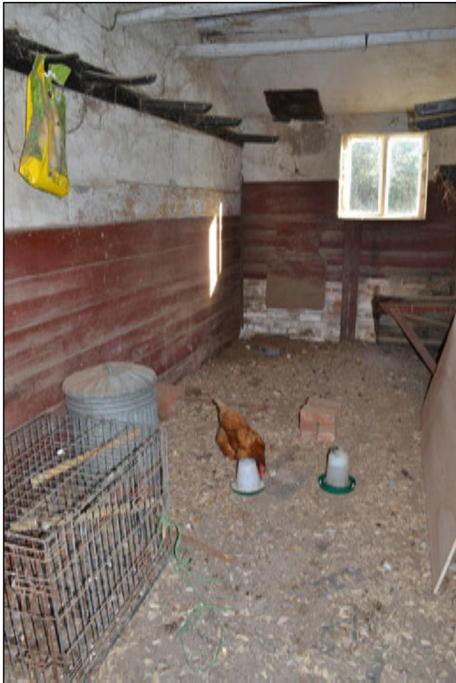
Figure 54: Tack room and store adjacent to the coal store and boiler room. The walls are lined with timber however parts of the plaster along the roof have been lost exposing timber laths beneath
