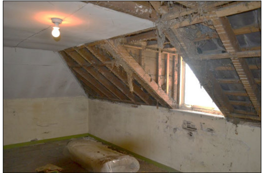
Figure 24: Attic room, note the exposed roof timbers and dormer window (right)
