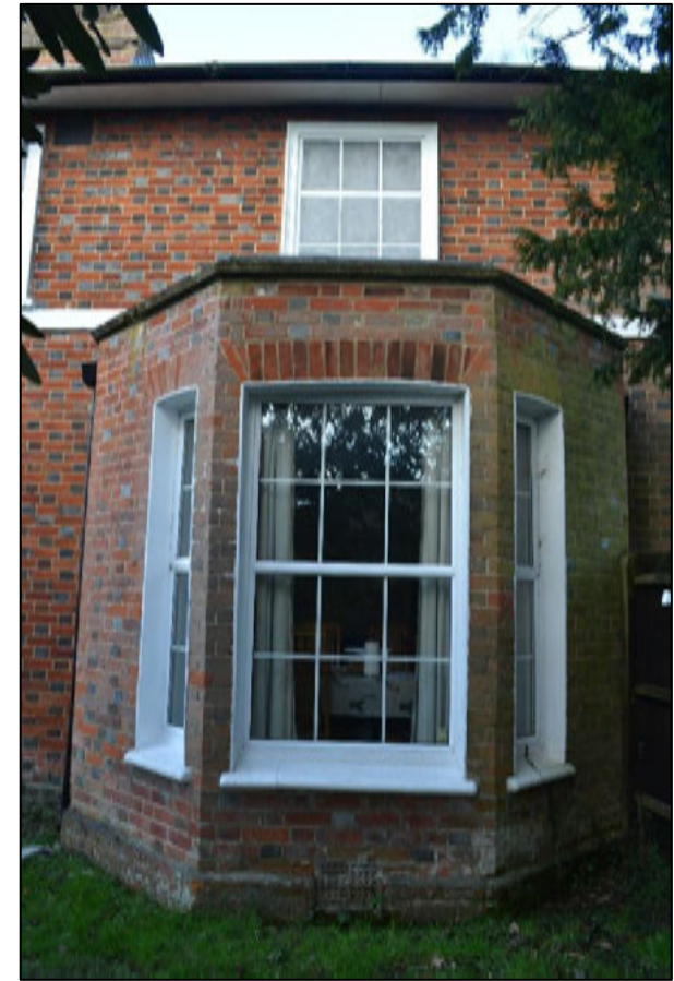
Figure 17: Details of the east elevation - note the painted blind windows on the first floor. The projecting bay window of the ground floor is thought to date from the late 19 th /early 20 th century
