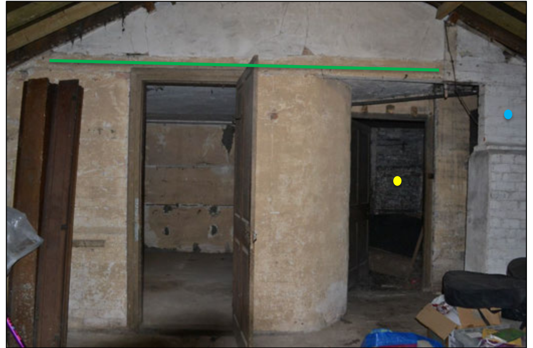
Figure 51: Further interior images of initial store - note the timber lintel highlighted in red indicating a potential former opening, the section of wall highlighted in green (which includes the curved wall) appears to be a later insertion and post-date the original masonry wall highlighted in blue, the coal store is highlighted in yellow.
