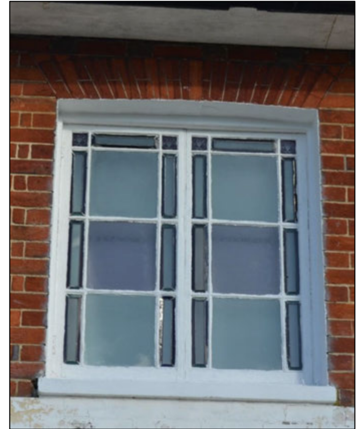
Figure 20 - Details of windows on the south elevation (left) inappropriate 20 th century uPVC top hung casement window, (centre) dormer window thought to originally house the clock when the house was briefly a school. (Right) Original timber single glazed leaded window - internally there is secondary glazing behind it. Note both windows (left and right) have flat segmental arches above
