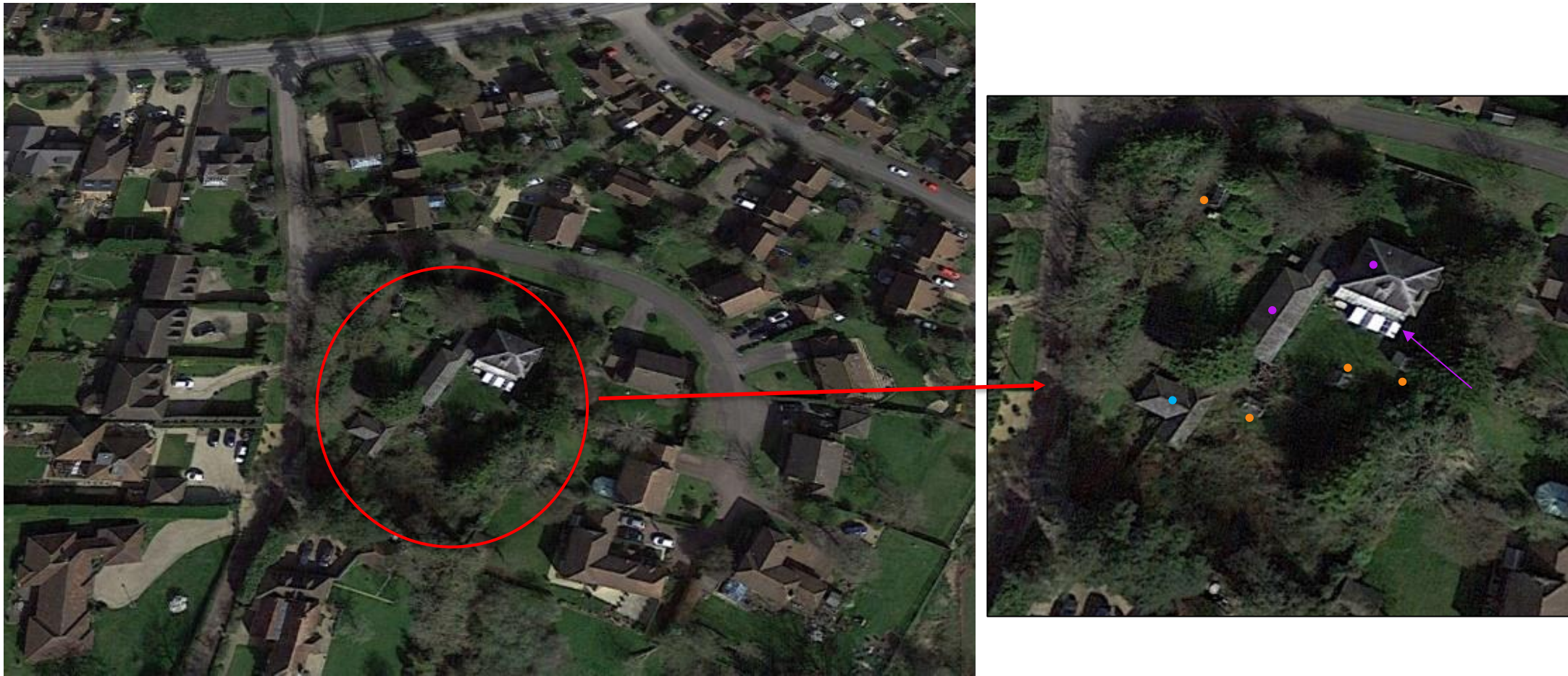
Figure 10: 2017 Google Aerial Image, approx. site location outlined in red Detail (right): Sussex Lodge and attached outbuilding highlighted in purple dot, detached stable/garage building highlighted in blue dot. Note the detached structure north of the stable/garage identified on the image above is gone, however there are a number of satellite structures within the garden (orange dots). The structure attached to the conservatory on the south elevation (purple arrow) has remained
