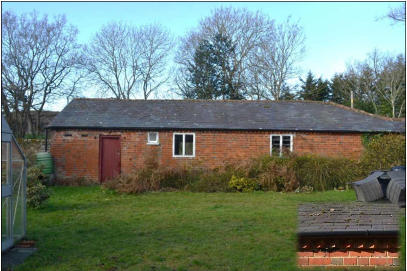
Figure 47: Eastern elevation of attached outbuilding (inset corbelling detail)
