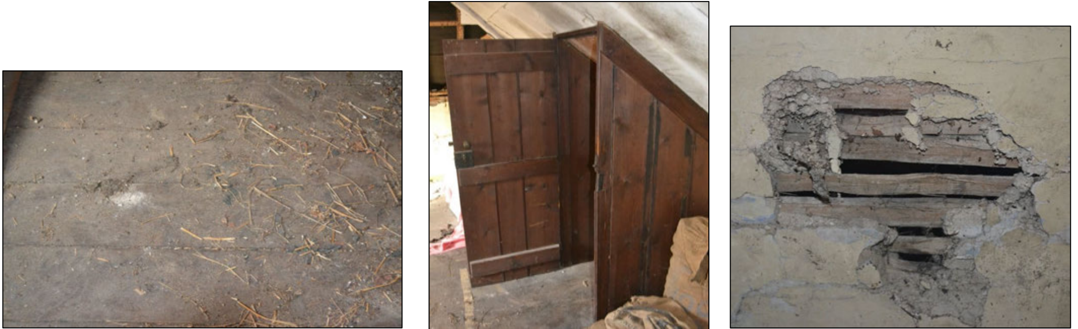
Figure 25: Attic room details (left) solid timber floor, (centre) timber door leading to stairs to access the ground floor, (right) exposed historic lath and plaster
