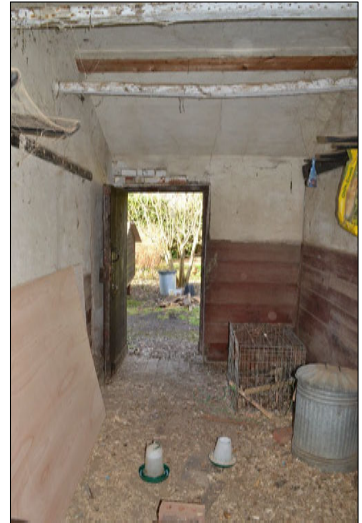
Figure 54: Tack room and store adjacent to the coal store and boiler room. The walls are lined with timber however parts of the plaster along the roof have been lost exposing timber laths beneath
