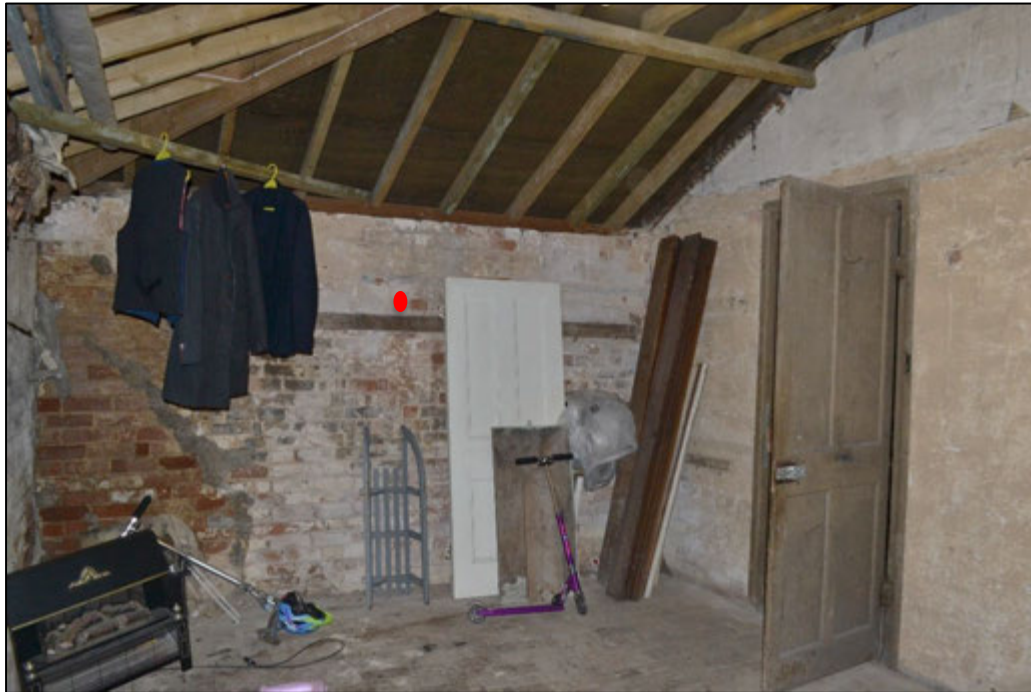
Figure 51: Further interior images of initial store - note the timber lintel highlighted in red indicating a potential former opening, the section of wall highlighted in green (which includes the curved wall) appears to be a later insertion and post-date the original masonry wall highlighted in blue, the coal store is highlighted in yellow.
