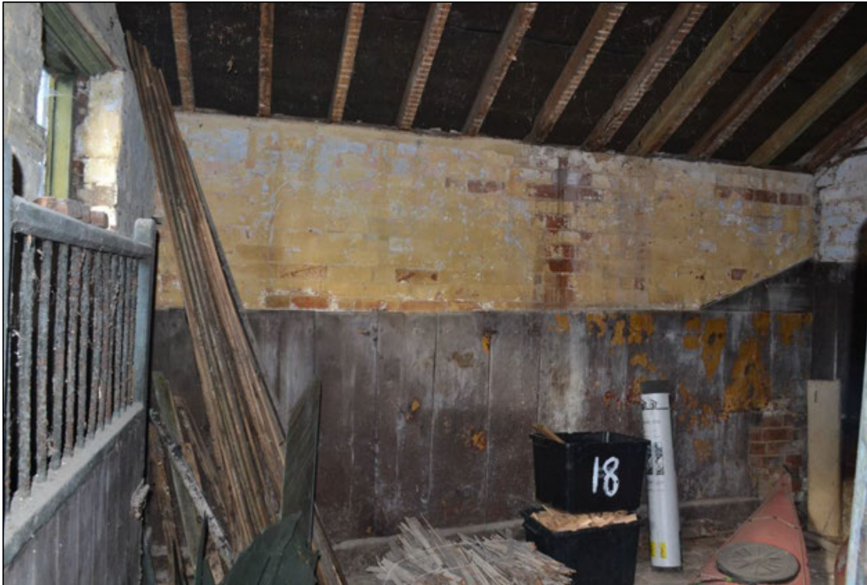
Figure 55: Final store room, now stable, (left) exposed roof timbers and bitumastic sarking felt, suggesting that the roof was last recovered in the late 1970s or 1980s. (Right) Evidence again of timber and brick stud wall separating the stable from the tack room
