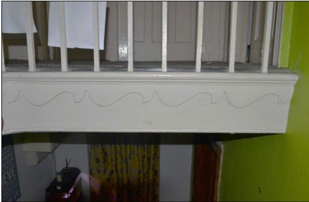
Figure 33 - Details of early 19 th century staircase, note the stick balusters, mahogany banister, and carved brackets under the treads
