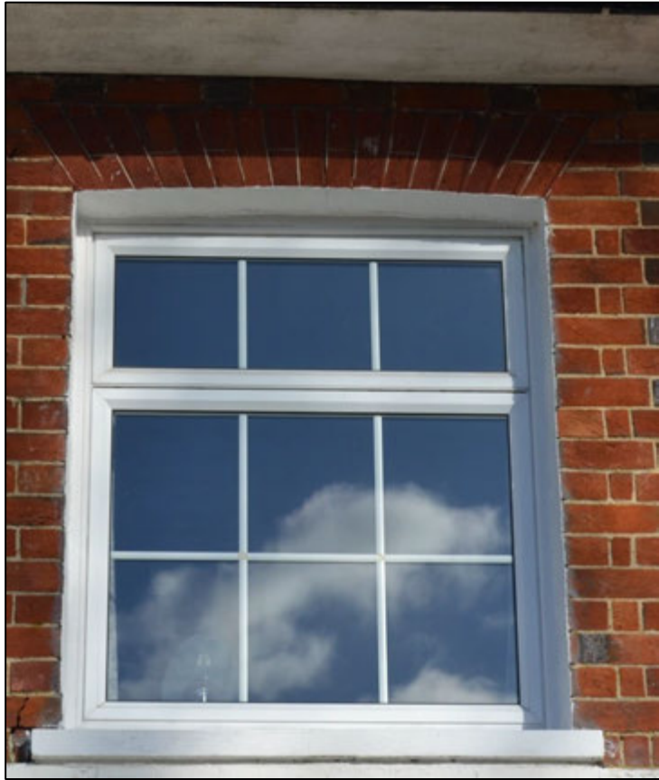
Figure 20 - Details of windows on the south elevation (left) inappropriate 20 th century uPVC top hung casement window, (centre) dormer window thought to originally house the clock when the house was briefly a school. (Right) Original timber single glazed leaded window - internally there is secondary glazing behind it. Note both windows (left and right) have flat segmental arches above
