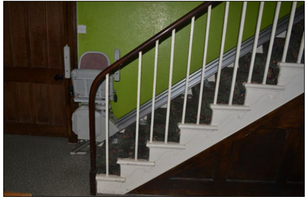
Figure 33 - Details of early 19 th century staircase, note the stick balusters, mahogany banister, and carved brackets under the treads
