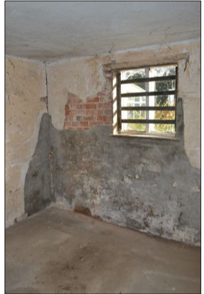
Figure 53: Internal view of boiler room- note (left) the evidence of the later timber frame and brick infill wall visible through the plaster/render. The concrete floor is a later 20 th century addition
