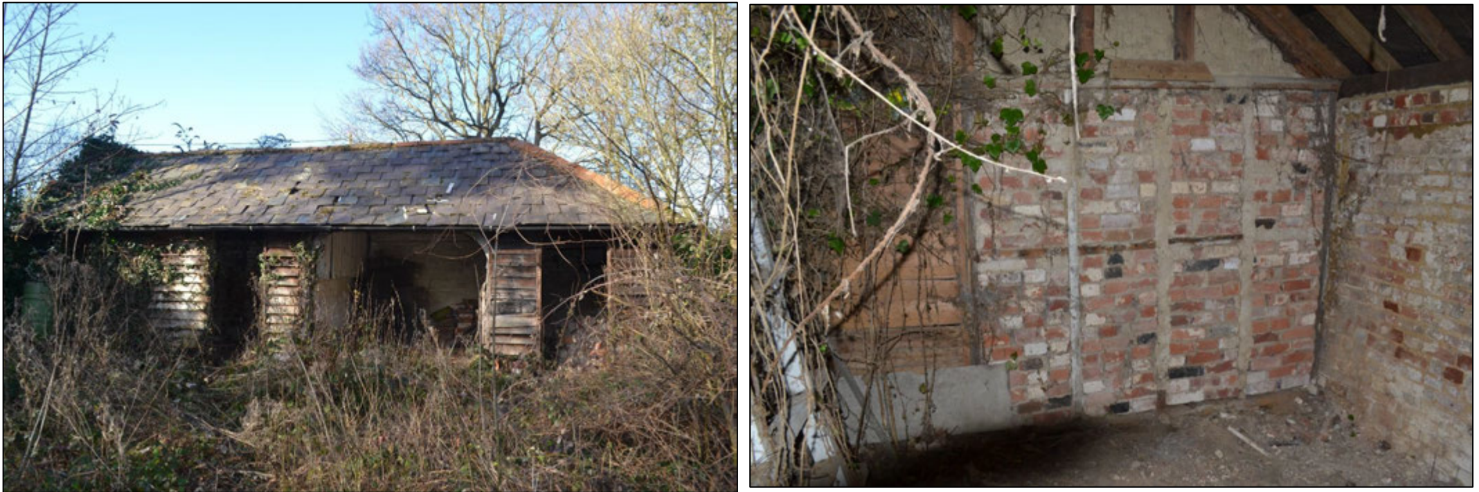
Figure 64: Historic outbuilding in south-west corner of the plot, (left) eastern elevation illustrating the various partitioned stables, (right) example of internal brick and timber partition wall
