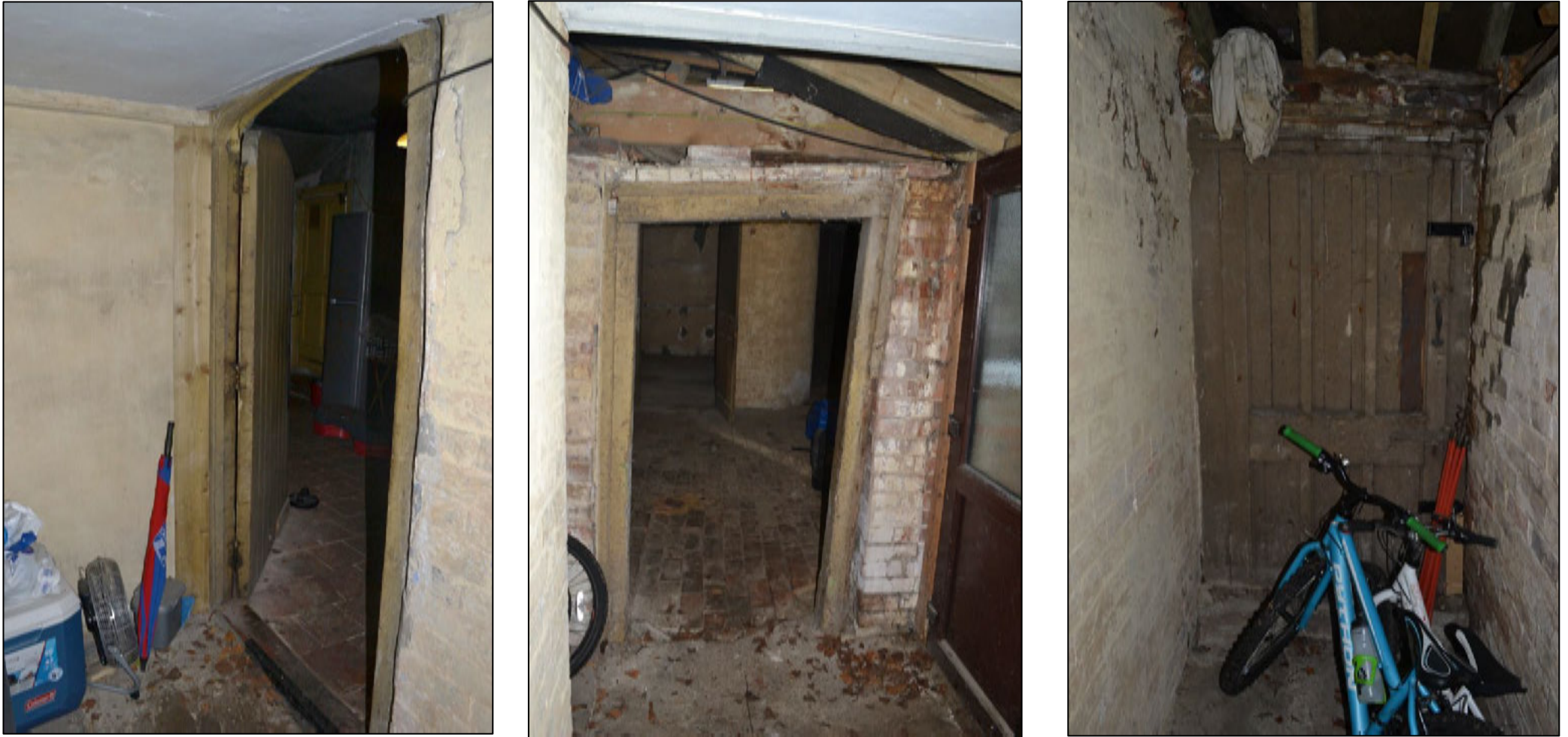
Figure 44: View inside later 20 th century extension that attaches the outbuilding to the principal house - (left) view of doorway taken from Arborfield Church, (centre) door way leading into outbuilding, (right) 19 th century door leading out into the southern garden at the rear of the property
