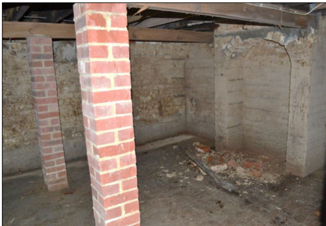
Figure 46: Cellar rooms - note the walls are brick lined and there are recessed oven arches
