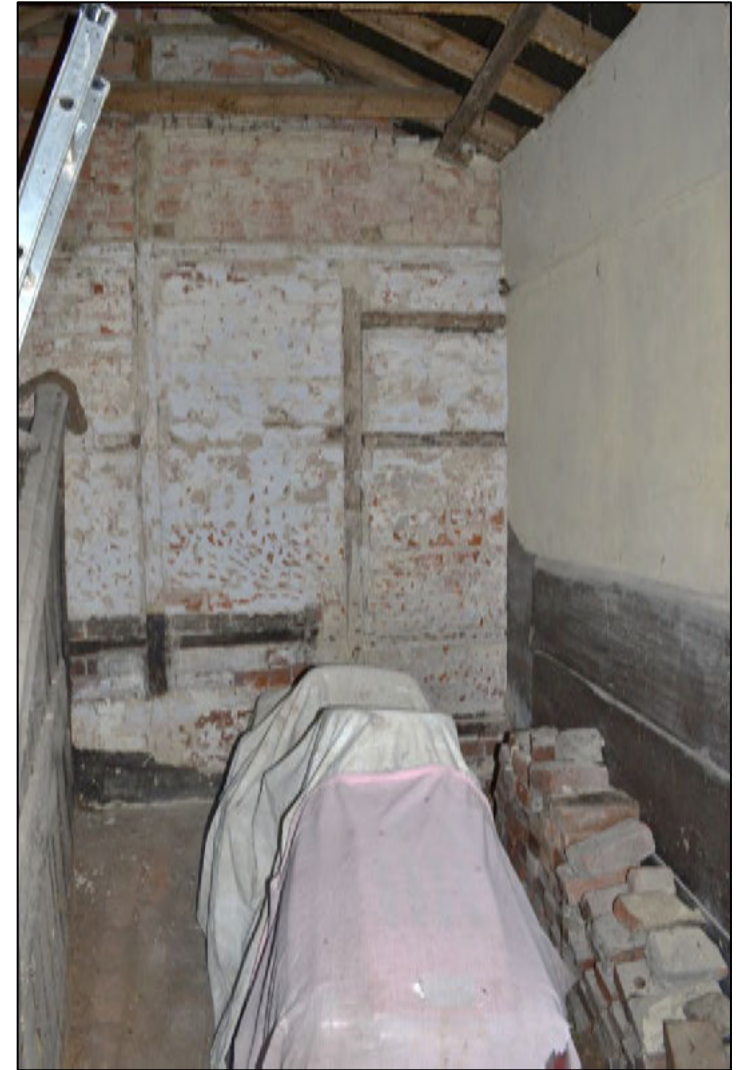
Figure 55: Final store room, now stable, (left) exposed roof timbers and bitumastic sarking felt, suggesting that the roof was last recovered in the late 1970s or 1980s. (Right) Evidence again of timber and brick stud wall separating the stable from the tack room
