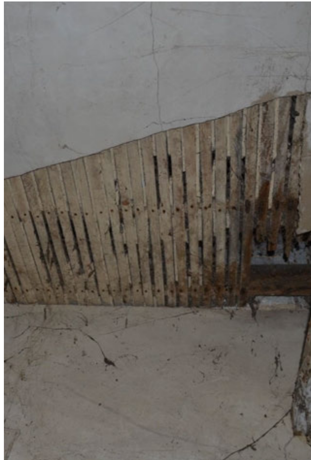
Figure 54: Tack room and store adjacent to the coal store and boiler room. The walls are lined with timber however parts of the plaster along the roof have been lost exposing timber laths beneath
