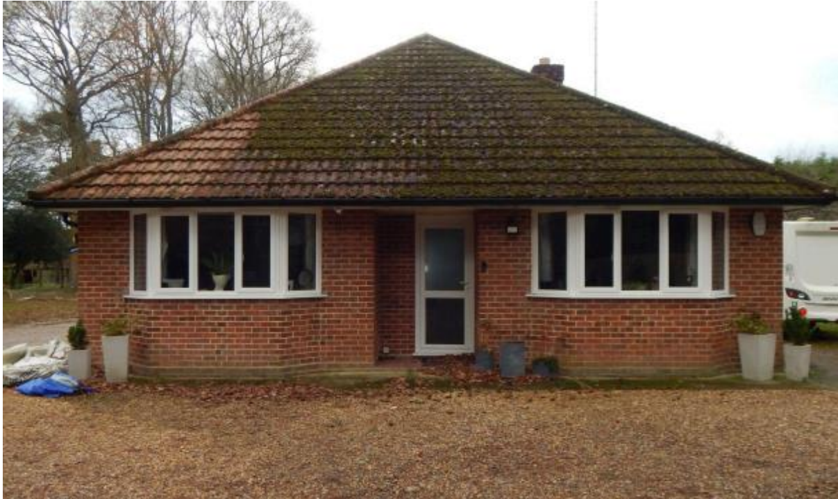
Image 1 – South facing elevation of the main dwelling
