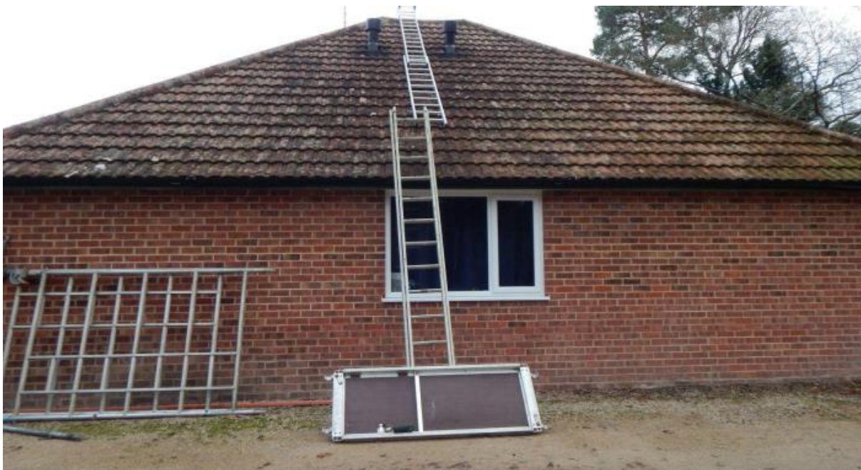
Image 4 – West facing elevation of the main dwelling
