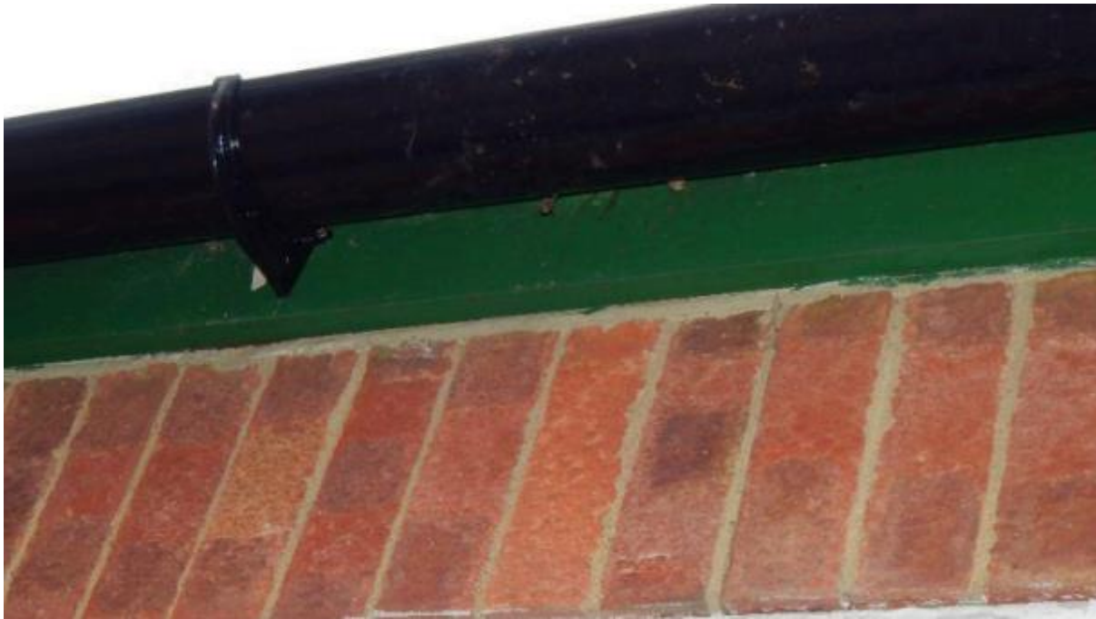
Image 14 – Facia coverings to the detached garage structure where no gaps or features of value to bats were observed
