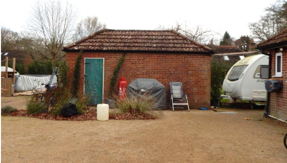
Image 12 – Detached garage structure located to the side of the main dwelling
