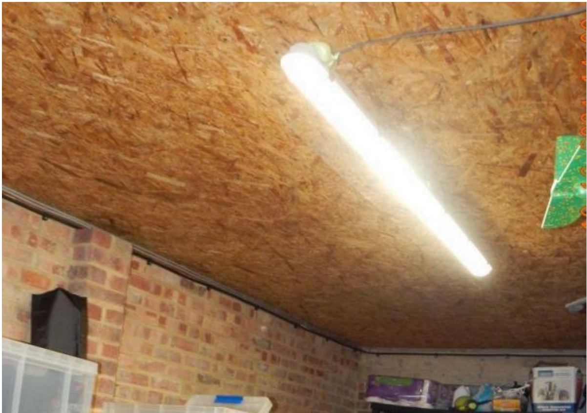
Image 15 – Internal view from below the roof coverings to the detached garage. No access available into the roof void spaces
