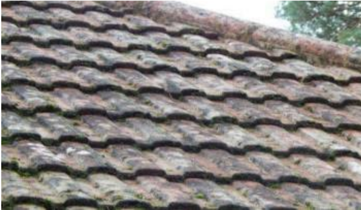
Image 5 – Close view of the main upper roof coverings to the main dwelling where no suitable features of value to bats were identified
