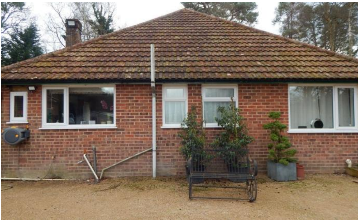
Image 2 – North facing elevation of the main dwelling
