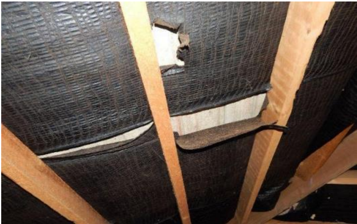
Image 9 – Internal view from within the main roof void spaces of the property
