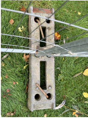
Protective Barrier (P.B.) (S.T.P.) Heras fencing panels, placed in rubber feet, which will be pinned to the ground using a soil pin. For impenetrable ground, the stabilisation bars will be mounted on a block to
