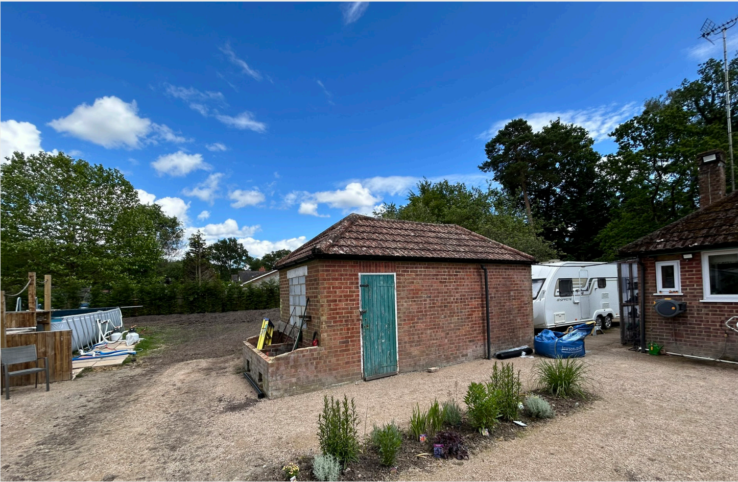
EXISTING PHOTO OF GARAGE TO BE DEMOLISHED
