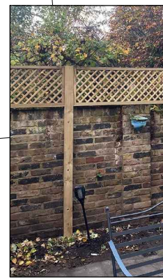
Timber Trellis Fence: 300mm high & timber posts
