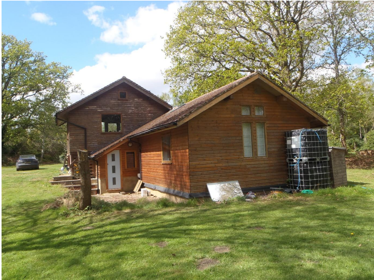
Photograph 3: showing a view of the building on the site (looking west)
