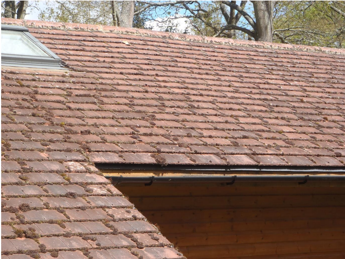
Photograph 4: showing a view of the roof of the building
