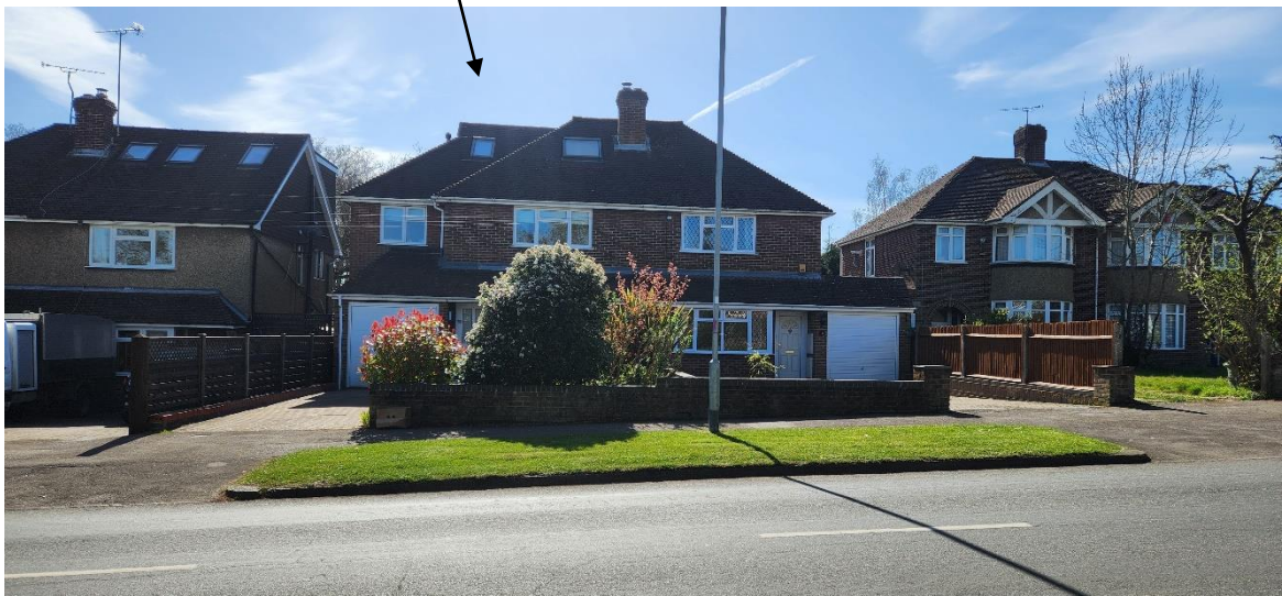
17 view of the neighbouring property No.24 with similar side extension
