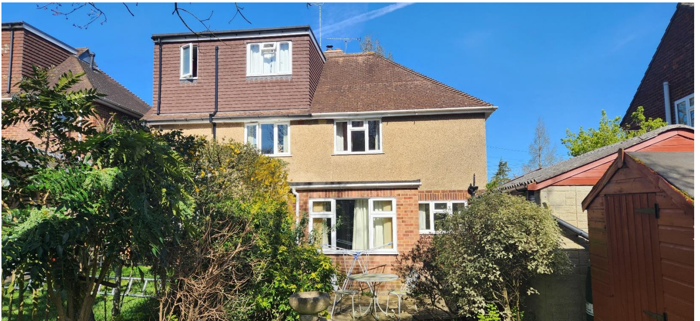
Existing rear view
