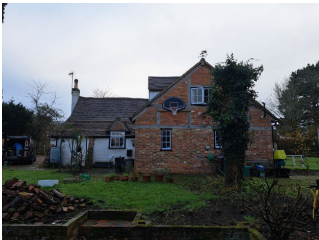
Photo 6 – View of rear (west) elevation
