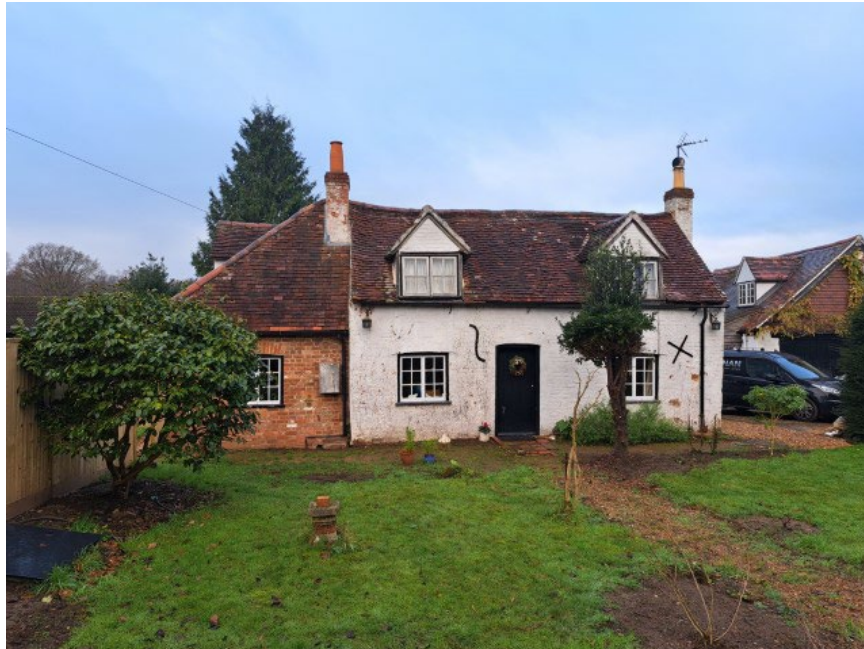
Photo 1 – View of the front (east) elevation
