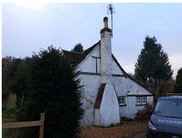
Photo 10 – View of side (north) elevation
