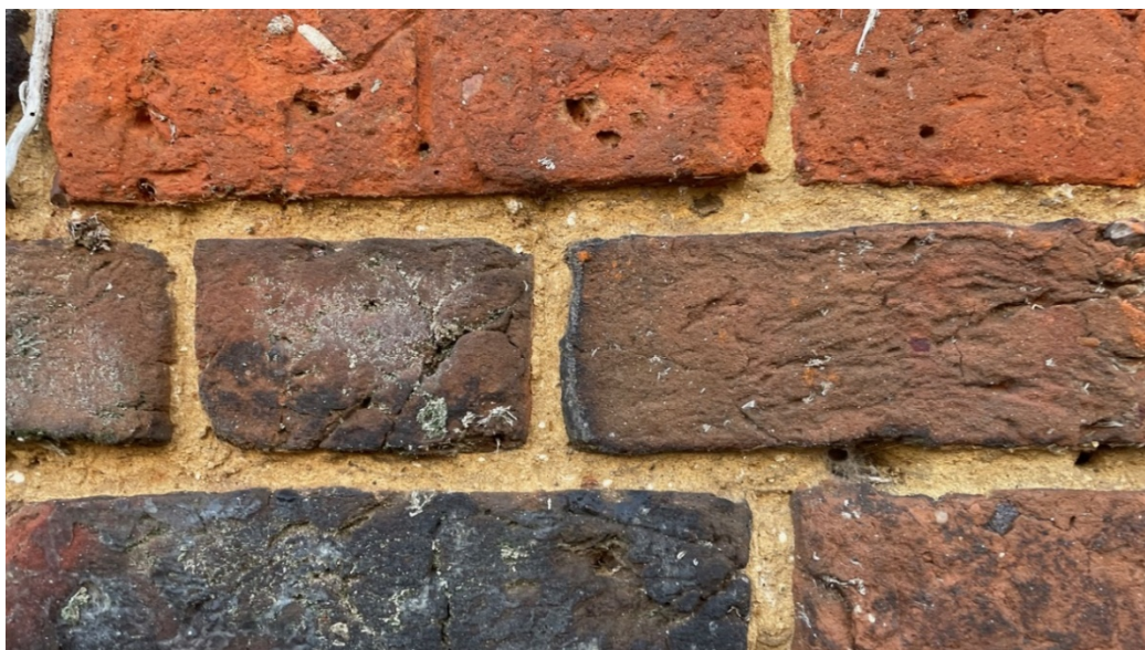
Sample mortar viewed against the existing H2 walling (11 th December 2025), which were still damp from recent rain.
