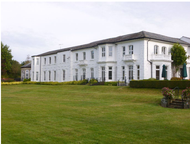
Plate 1: West elevation of Thamesfield
