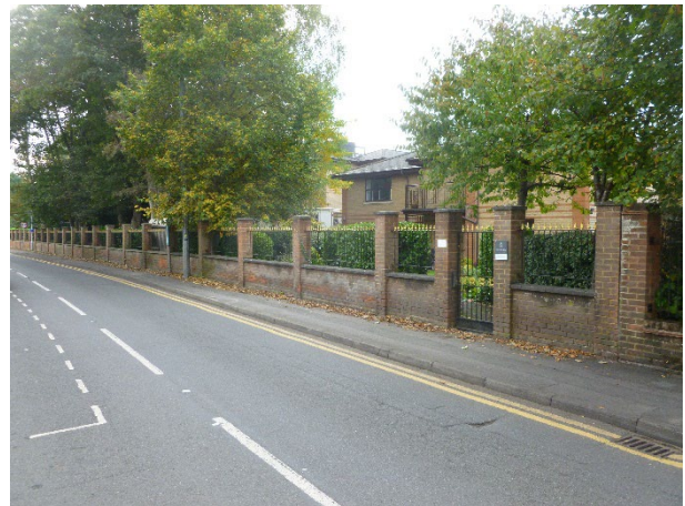
Plate 10: The Site from Wargrave Road, facing south
