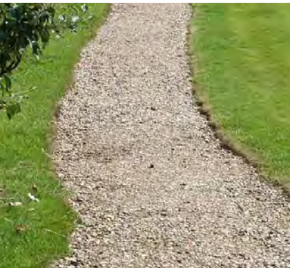
SELF-BINDING GRAVEL FOOTPATH
