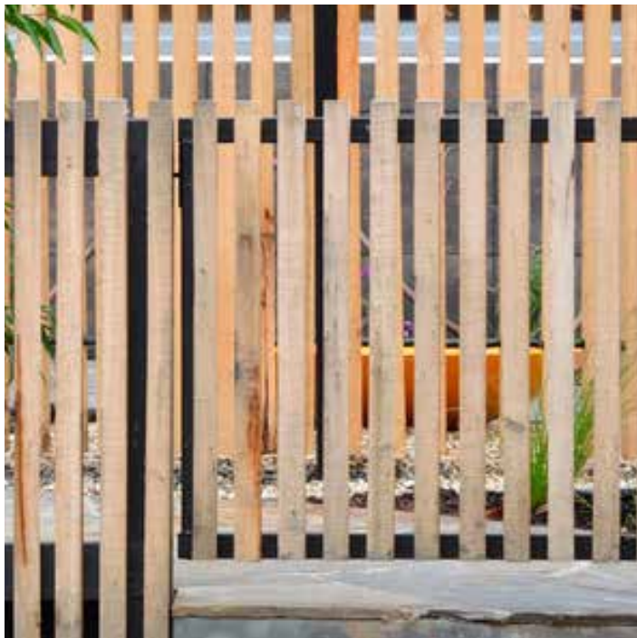
Vertical timber clad fencing to the cycle enclosure
