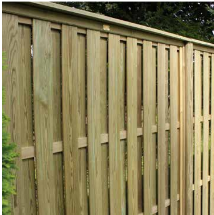
Vertical timber hit and miss fencing to the southern site boundary
