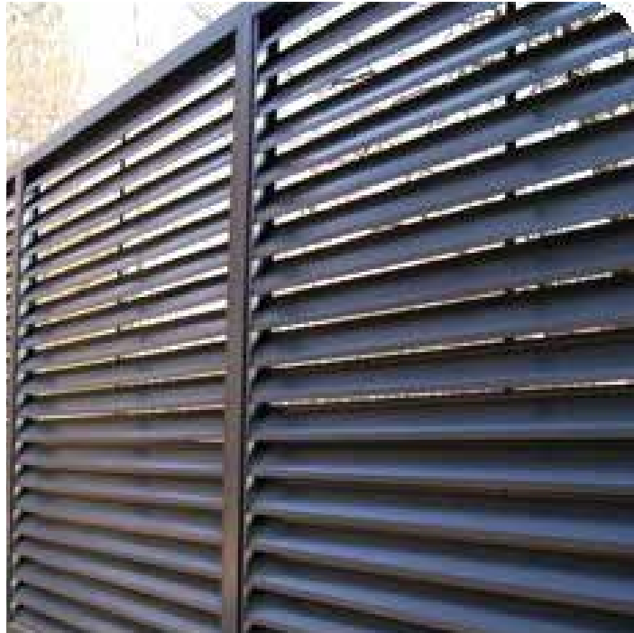
Louvred enclosure to rooftop plant areas to reduce aesthetic and acoustic impact
