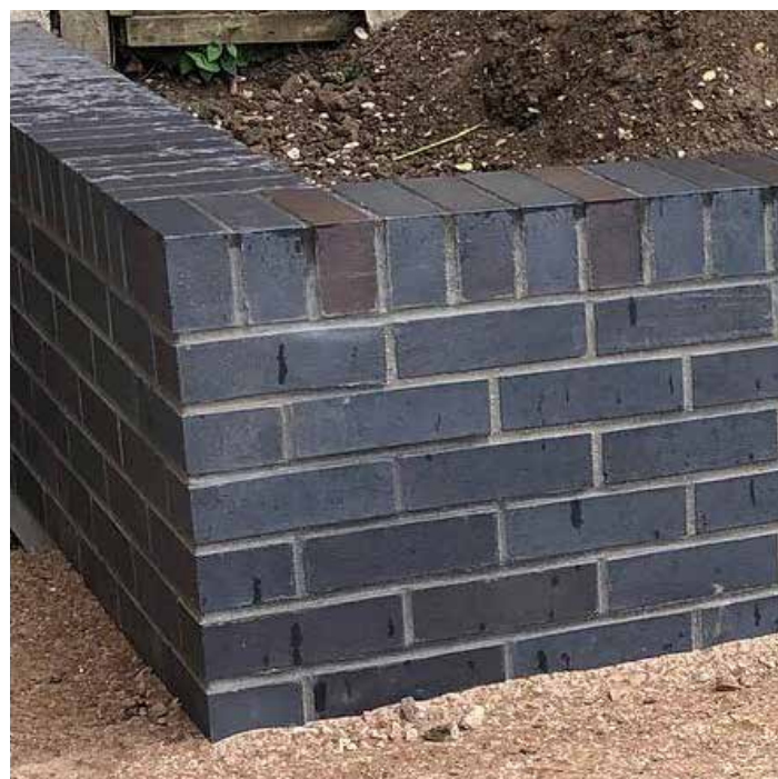
Blue engineering brick to planters
