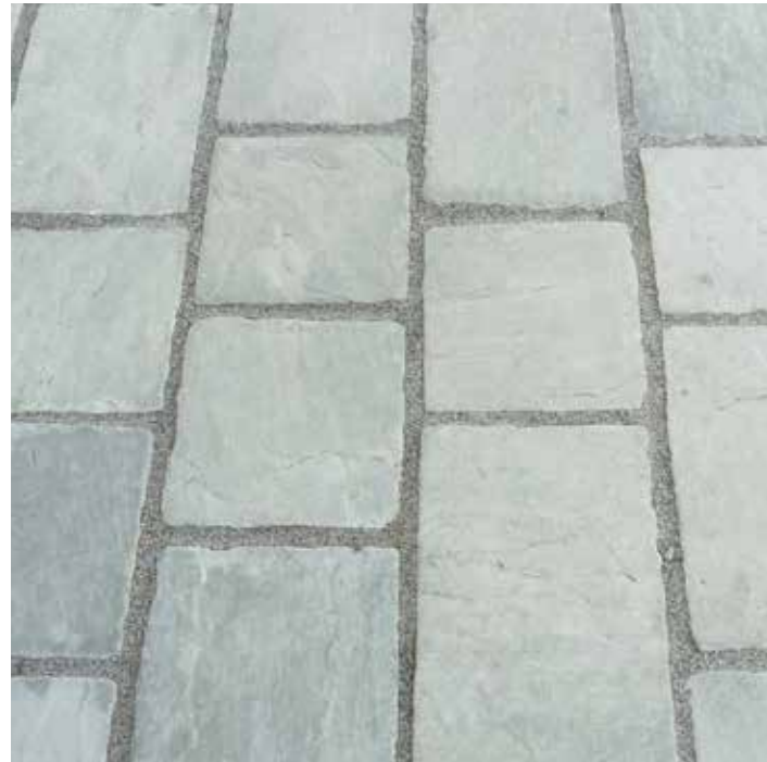
Grey sett paving stones in light grey to provide contrasting parking demarcation
