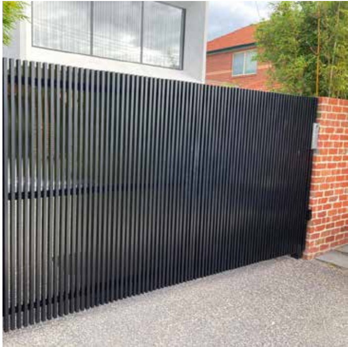
Dark grey, vertically clad metal pedestrian and vehicle gates to the western site boundary
