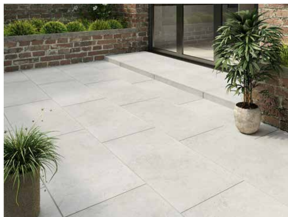
Light grey external porcelain paving to the pedestrian areas
