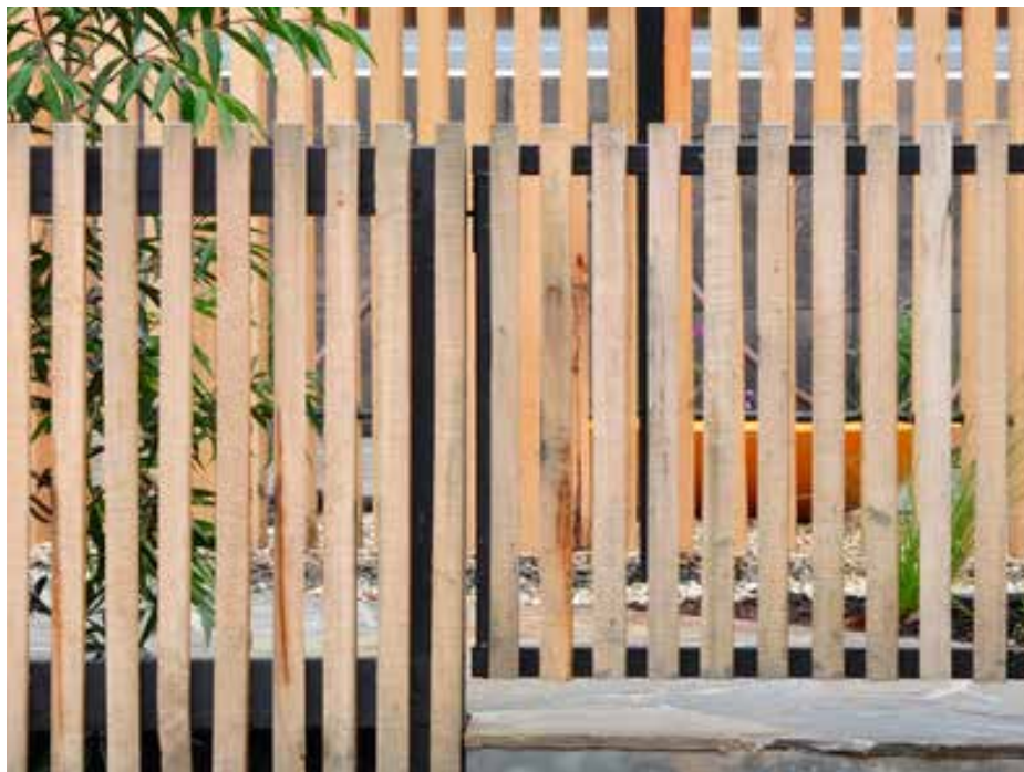
Vertical timber clad fencing to the cycle enclosure
