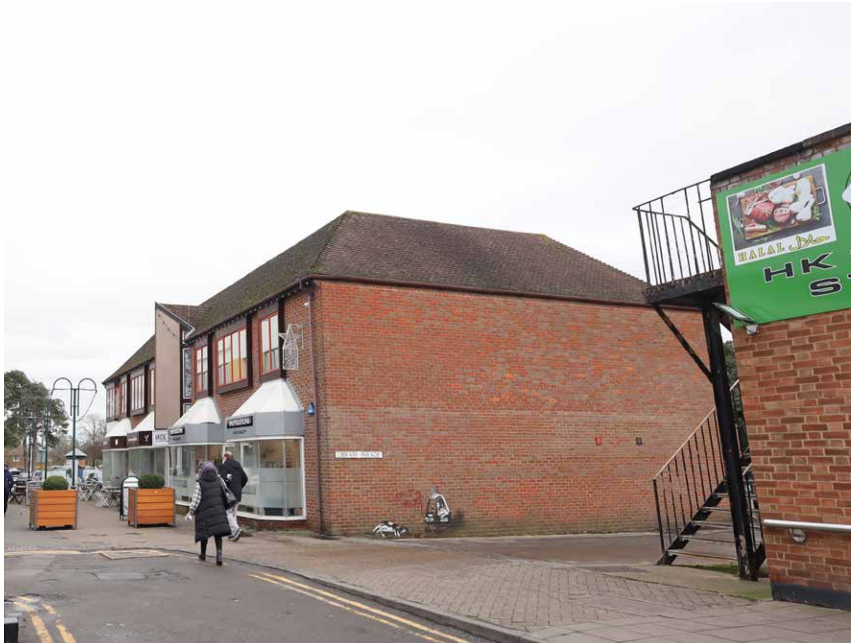
Existing view looking east through Library Parade
