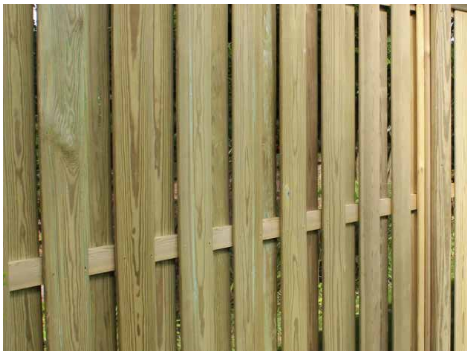
Vertical timber hit and miss fencing to the southern site boundary
