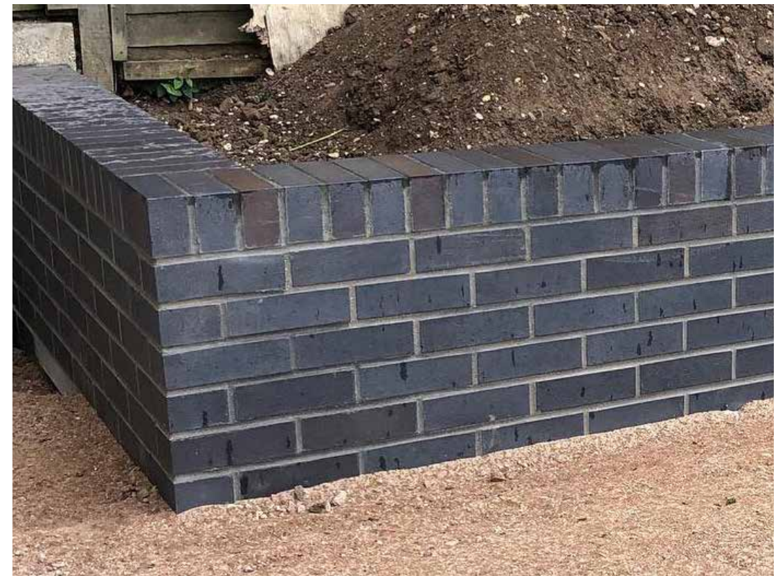
Blue engineering brick planters to the south, west and east boundary lines
