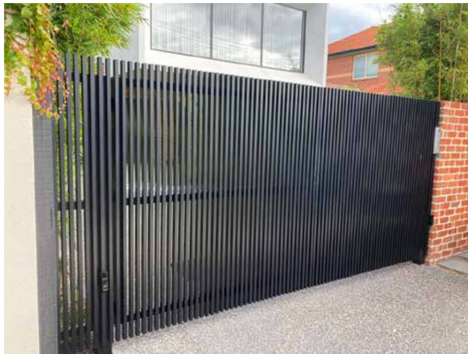
Dark grey, vertically clad metal pedestrian and vehicle gate to the western site boundary
