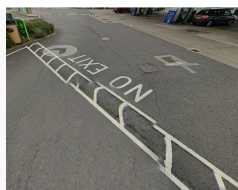
Ref #33.1 - Speed ramp to site entrance from A4 London Road
