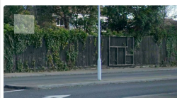
Ref #26.1 - Wooden fence on boundary line behind proposed EV charging area
