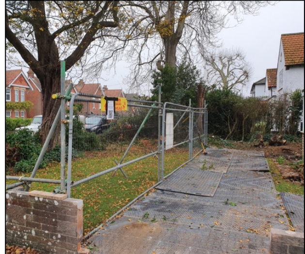
GP2: Tree protection barriers & trackmat ground protection
