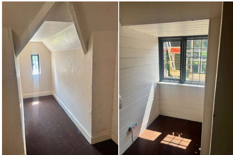
Figure 4: Internal photos showing limited scope to insulate below rafter levels in dormers and sloping ceilings due to potential to limit head room
