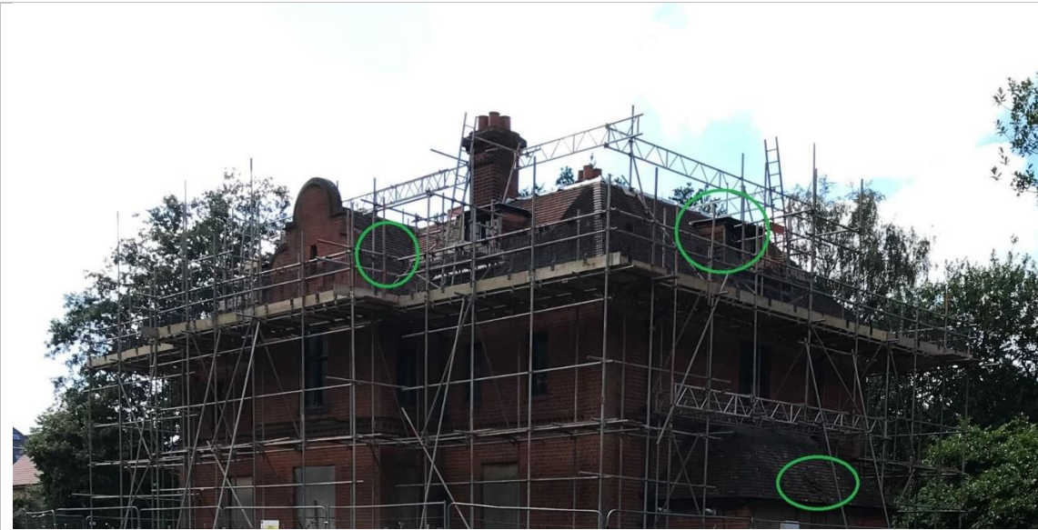
Photo 10. Potential roost features at the Moat House
