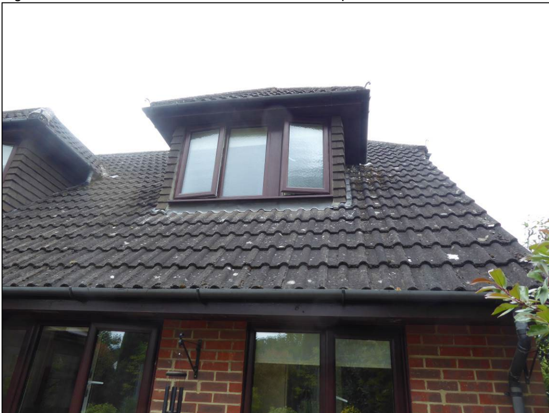
Figure 9. Dormer windows. 23b Pine Drive, Finchampstead, 02.07.24
