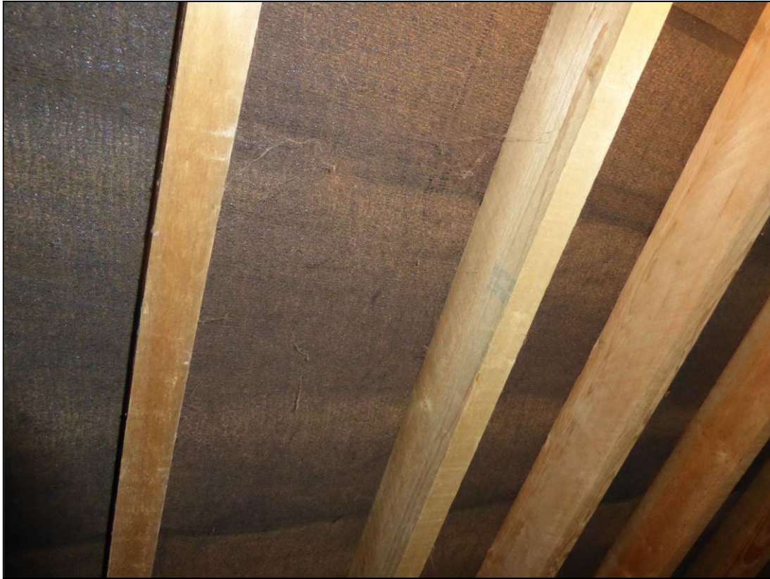
Figure 15. Example of bitumen lining. 23b Pine Drive, Finchampstead, 02.07.24
