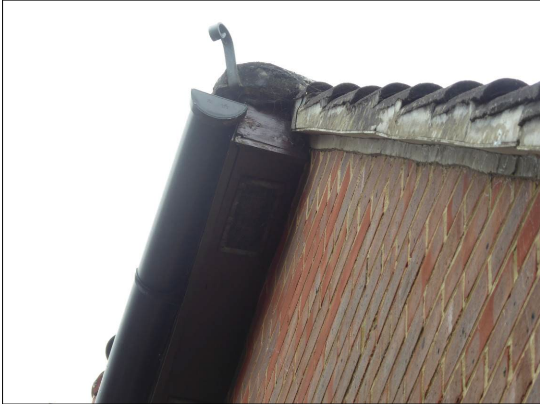
Figure 8. Example of soffits and fascias. 23b Pine Drive, Finchampstead, 02.07.24
