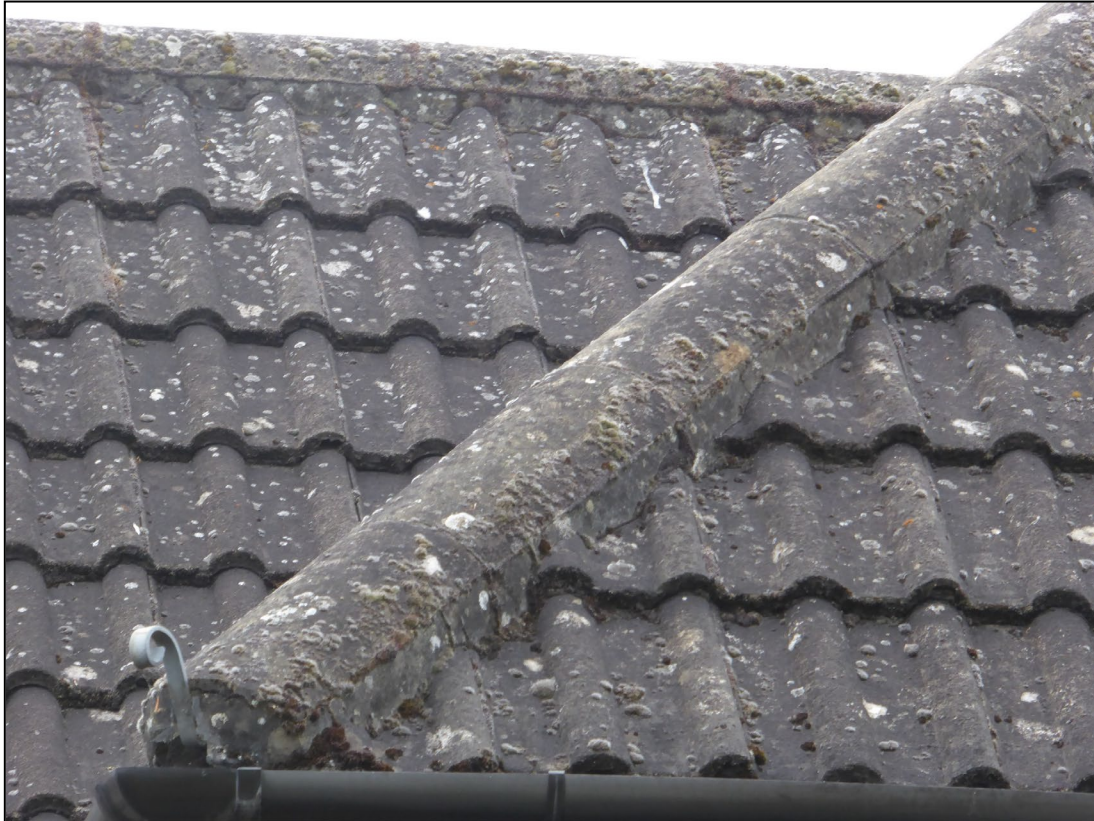
Figure 6. Tightly fitted hip tiles. 23b Pine Drive, Finchampstead, 02.07.24
