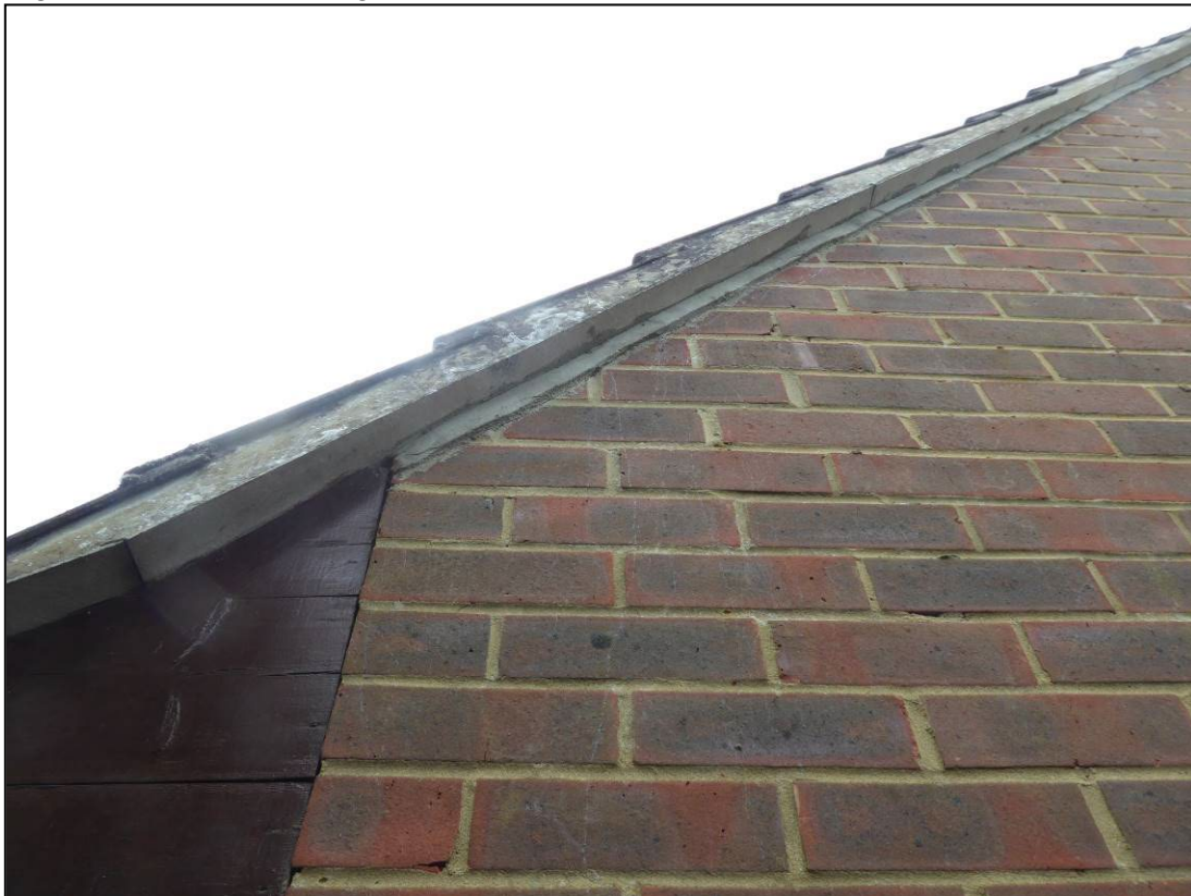
Figure 7. Example of verges. 23b Pine Drive, Finchampstead, 02.07.24
