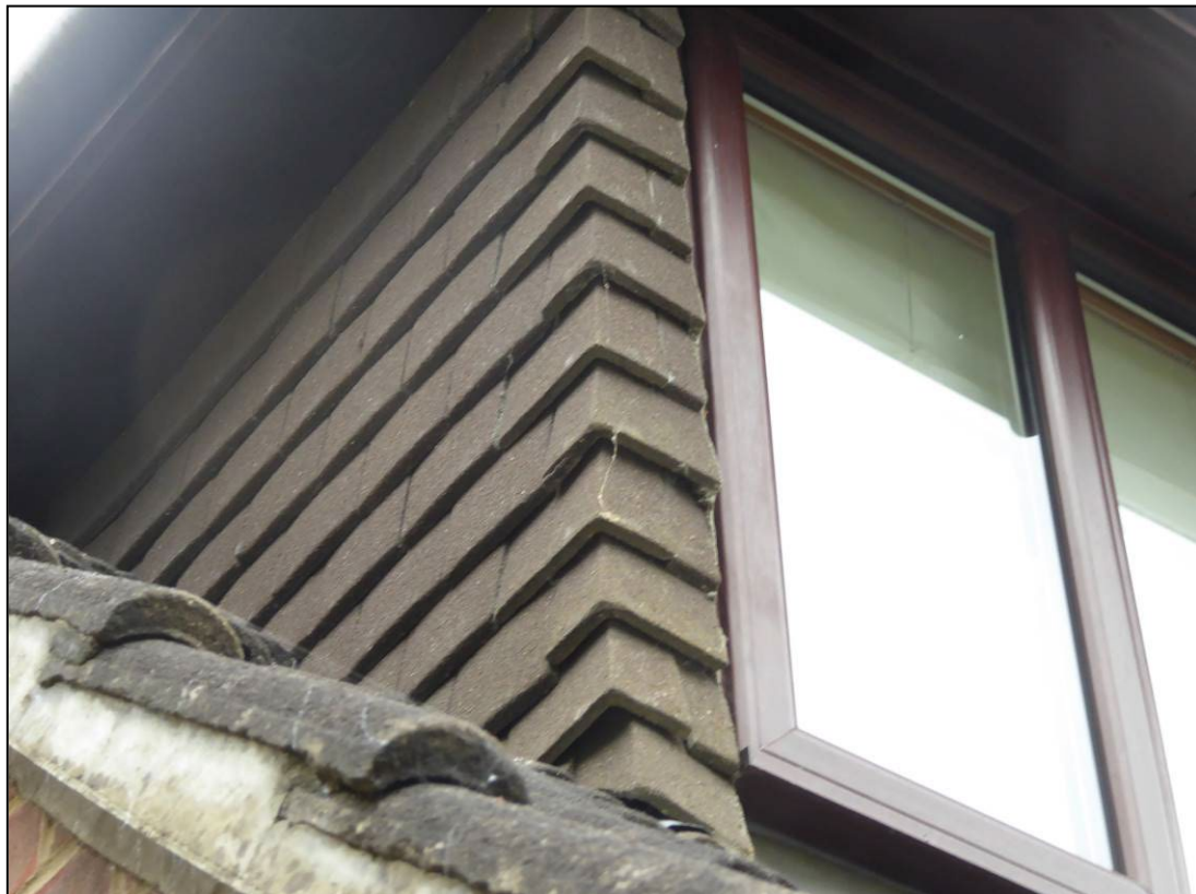
Figure 11. Hanging tiles on dormer windows. 23b Pine Drive, Finchampstead, 02.07.24
