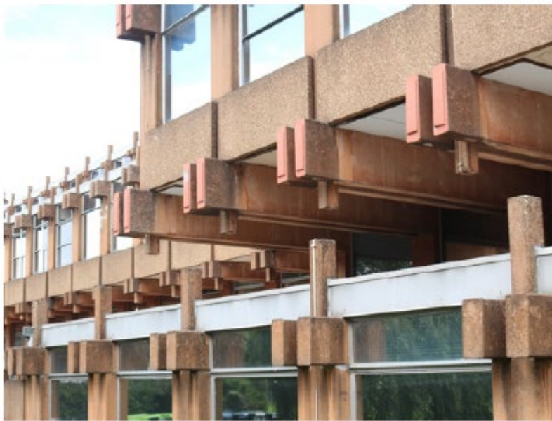
Standard beams (below) and post-tensioned beams, distinguished by the infilled anchorage pockets (above)
