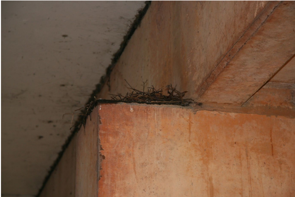
Example of bird's nest to undercroft beams
