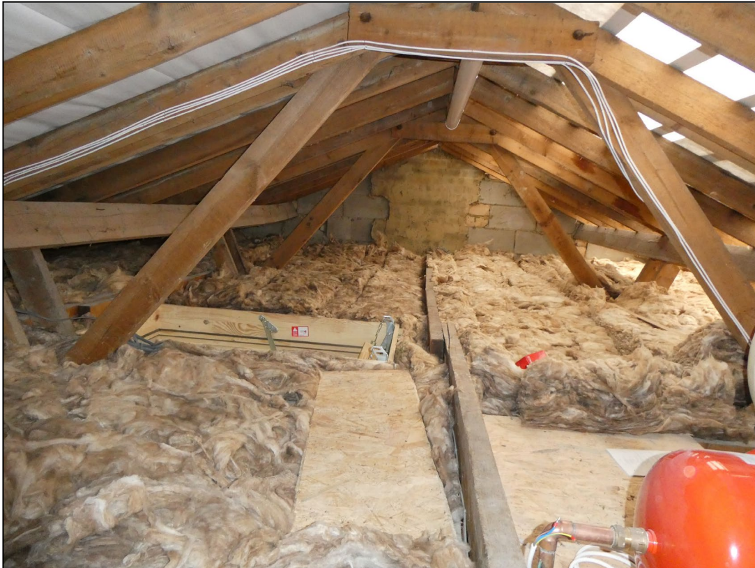
Figure 8. Example main loft space and membrane lining. 82 Wargrave Road, Twyford. 27.05.25
