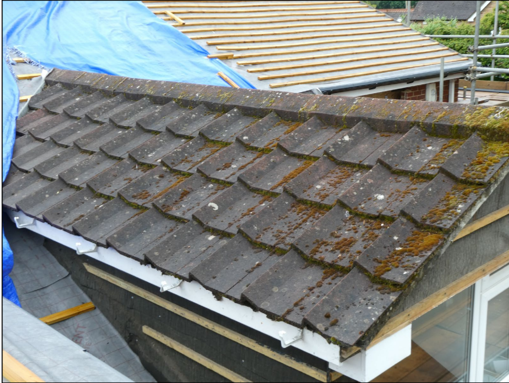
Figure 6. Example sealed roof and ridge tiles on dormer. 82 Wargrave Road, Twyford. 27.05.25
