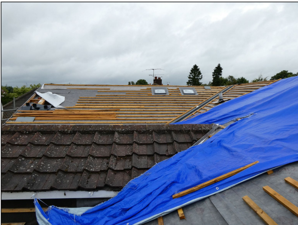
Figure 5. Example untiled and tarpaulined section of roof. 82 Wargrave Road, Twyford. 27.05.25
