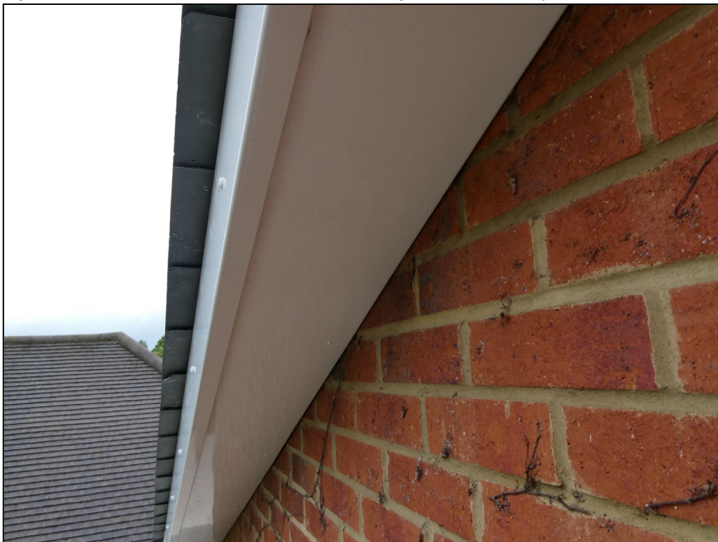
Figure 7. Sealed soffits and fascias. 82 Wargrave Road, Twyford. 27.05.25
