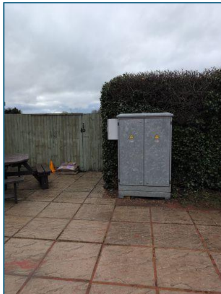
Upto 0.5m of hedge removed to allow construction, protective fencing to be installed during construction to protect retained hedge.
