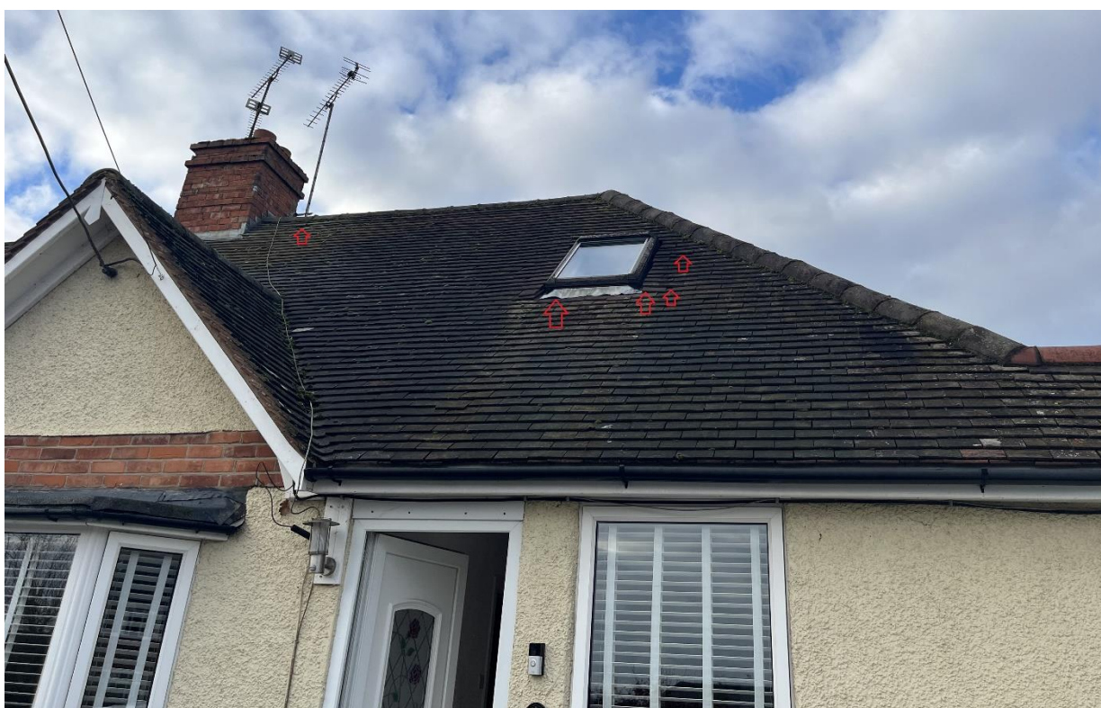
Figure 3. East elevations looking west: Red arrows indicate potential openings for crevice roosting bats.
