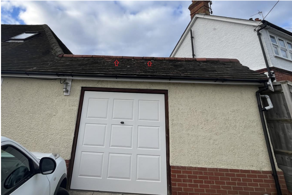
Figure 4. East elevations of garage looking west: Red arrows indicate potential openings for crevice roosting bats.
