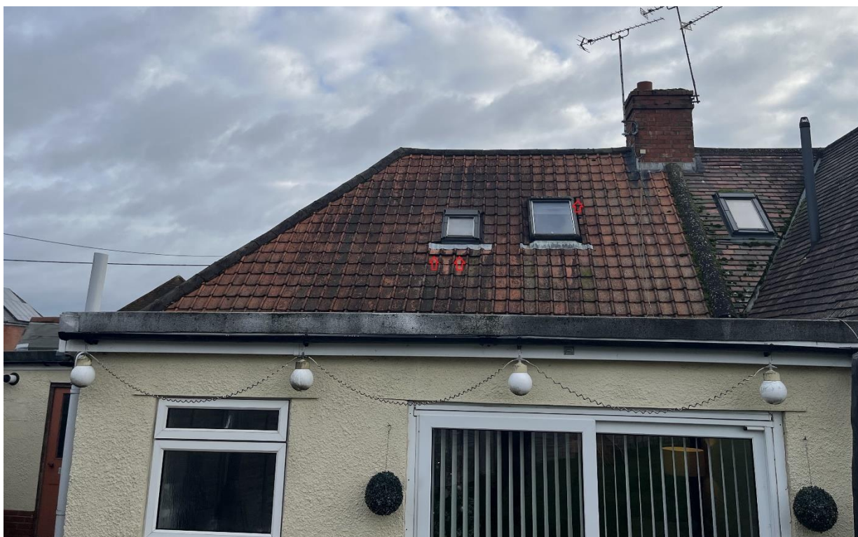
Figure 2. West elevations looking east: Red arrows indicate potential openings for crevice roosting bats.
