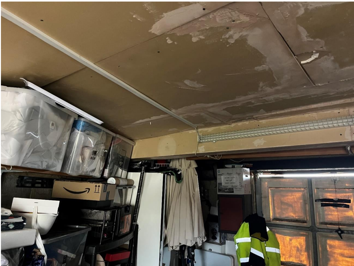
Figure 5. Garage interior looking northeast
