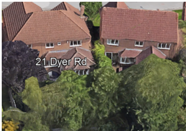
Figure 2 - screenshot showing no. 21 Dyer Road on the left and no. 19 Dyer Road on the right. This shows the distance between the two properties and how no. 19 sits back from no. 21. The window on the left-hand side of no. 19 is where the vertical loss of light test was taken from.
