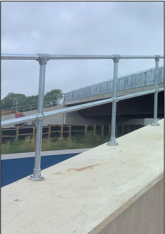
DETAIL 10 - GUARD RAIL ON WINGWALLS (SEE NOTE 4)
