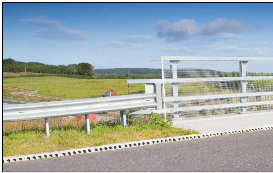
DETAIL 1 - PARAPET TO SAFETY BARRIER TRANSITION
