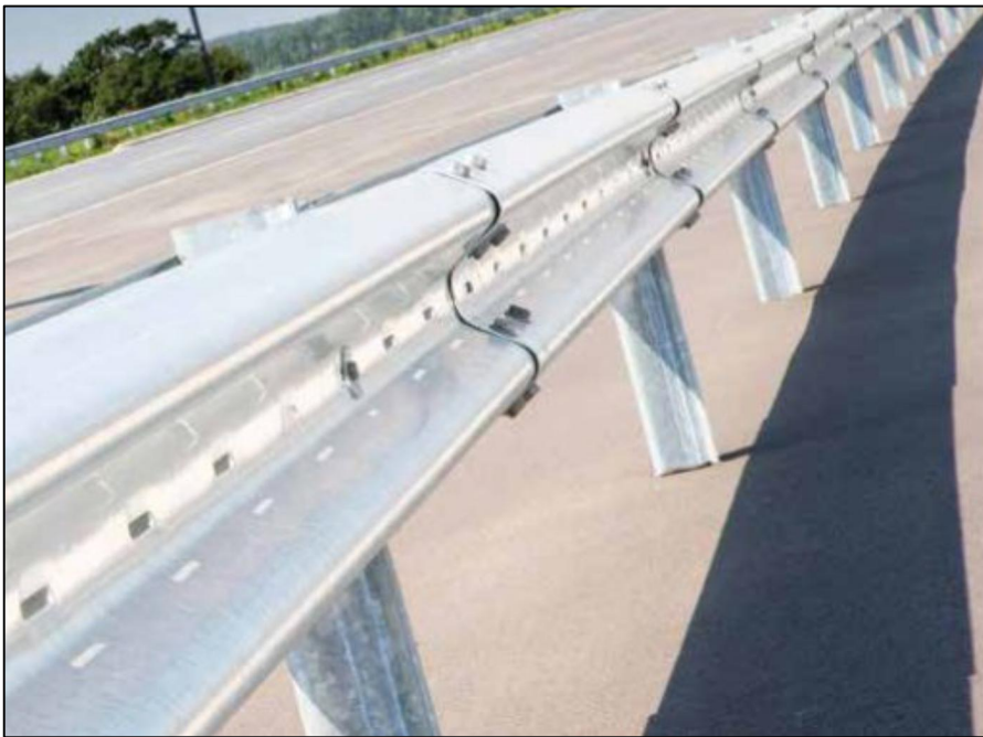
DETAIL 2 - SAFETY BARRIER
