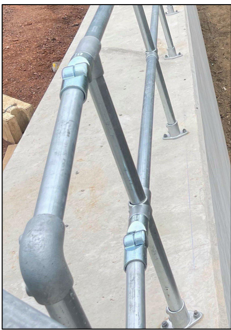
DETAIL 9 - GUARD RAIL ON WINGWALLS (SEE NOTE 4)
