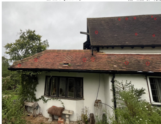
Figure 4. Southern elevations (western half) looking north. Red arrows indicate potential openings for crevice roosting bats.
