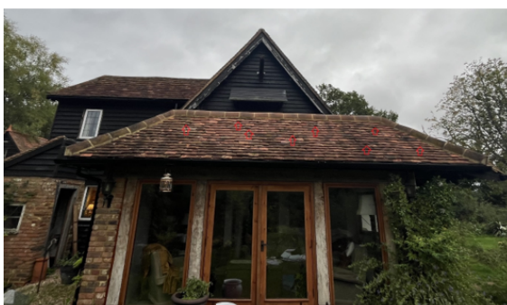
Figure 5. Western elevations looking east. Red arrows indicate potential openings for crevice roosting bats.
