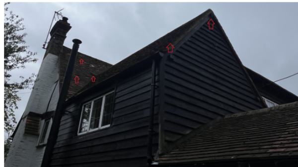
Figure 6. Northern and eastern elevations looking south. Red arrows indicate potential openings for crevice roosting bats.
