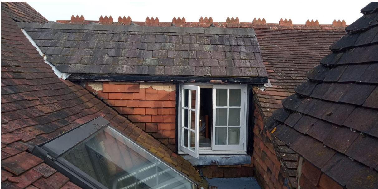
Photo E: mansard roof with section of slate tiles
