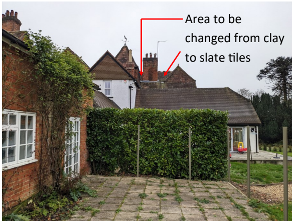
Photo C: view from the garden looking south-east
