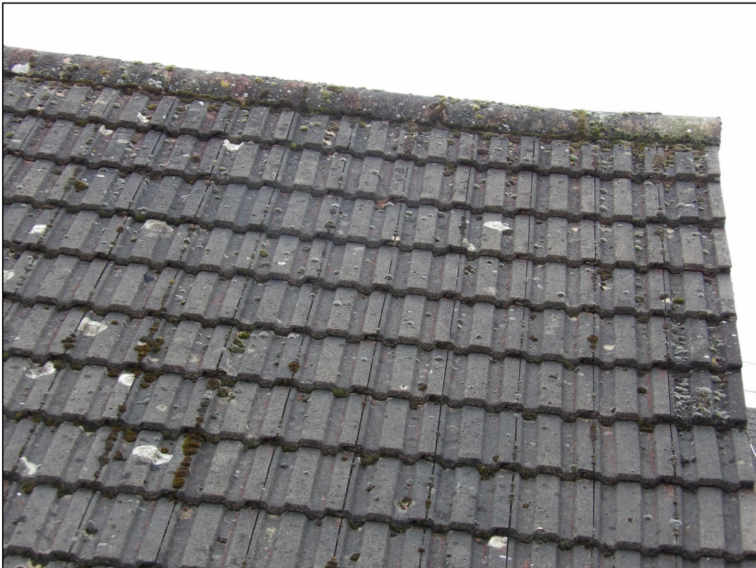
Figure 4. Tightly fitted roof and ridge tiles. 44 Cutbush Lane, Shinfield. 04.03.26
