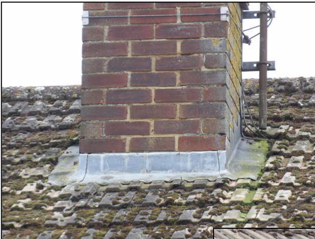
Figure 6. Example flush lead flashing. 44 Cutbush Lane, Shinfield. 04.03.26
