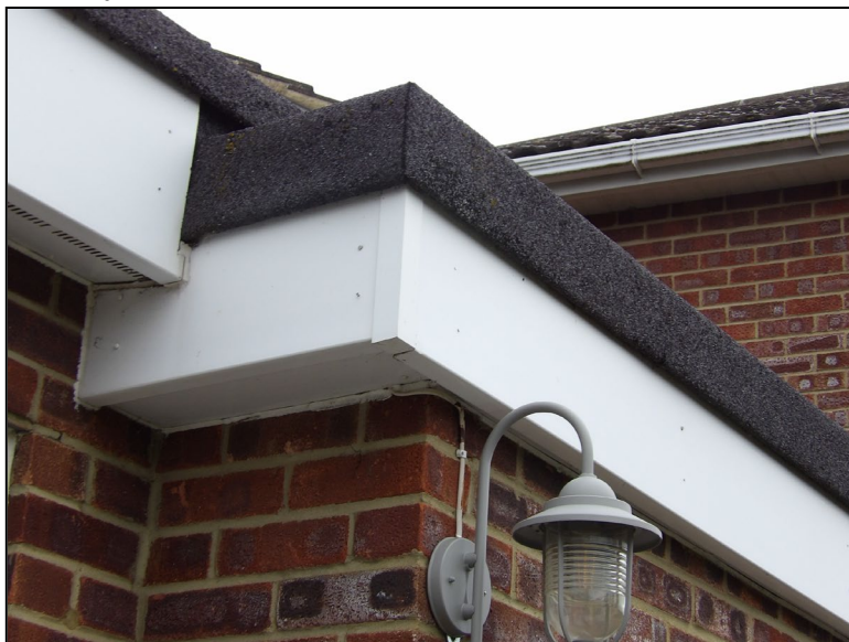
Figure 10. Example sealed uPVC soffits and fascias on single storey sections of the property. 44 Cutbush Lane, Shinfield. 04.03.26
