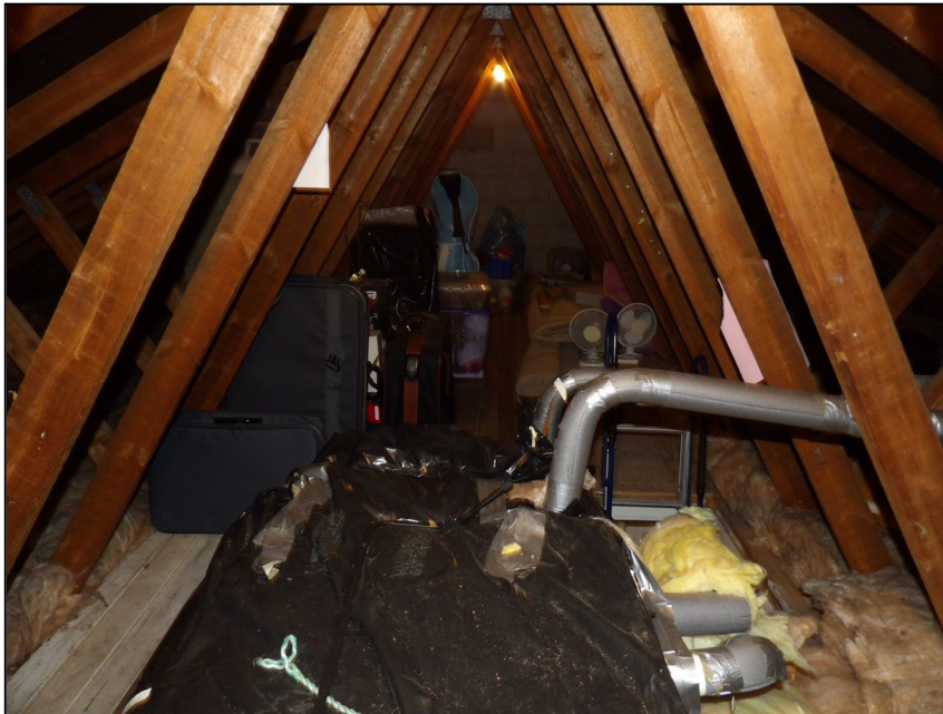
Figure 11. Example of loft space. 44 Cutbush Lane, Shinfield. 04.03.26
