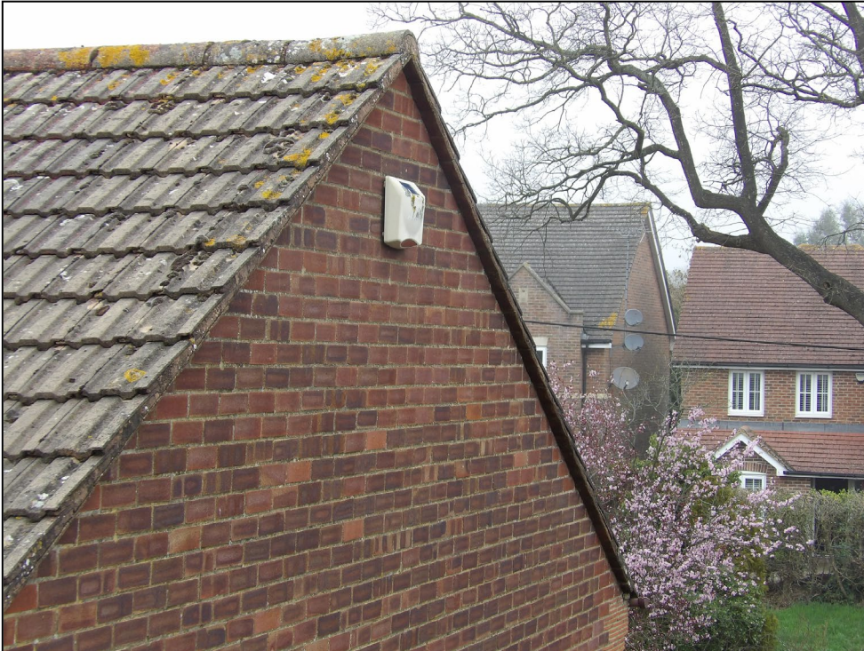
Figure 5. Example of sealed verges. 44 Cutbush Lane, Shinfield. 04.03.26
