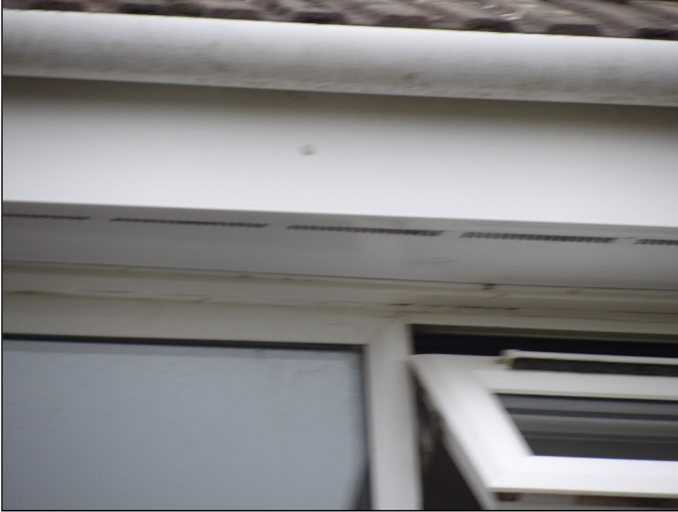
Figure 7. Example sealed uPVC soffits and fascias. 44 Cutbush Lane, Shinfield. 04.03.26
