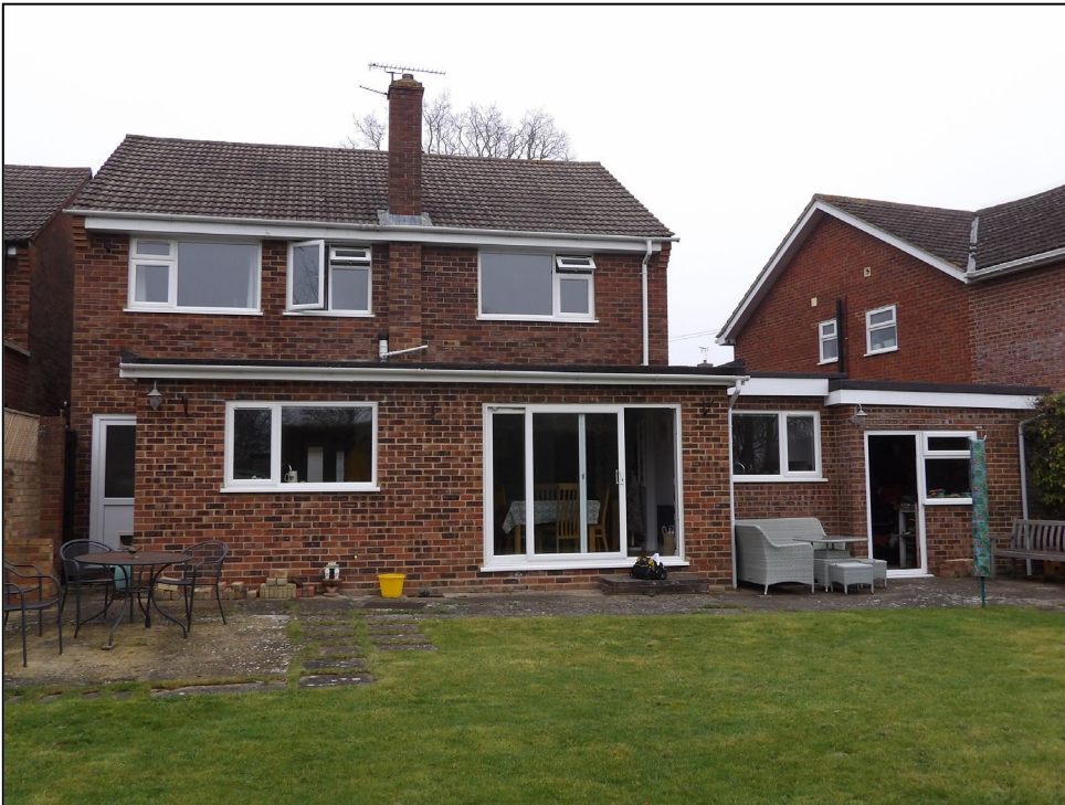
Figure 8. Rear view of property. 44 Cutbush Lane, Shinfield. 04.03.26
