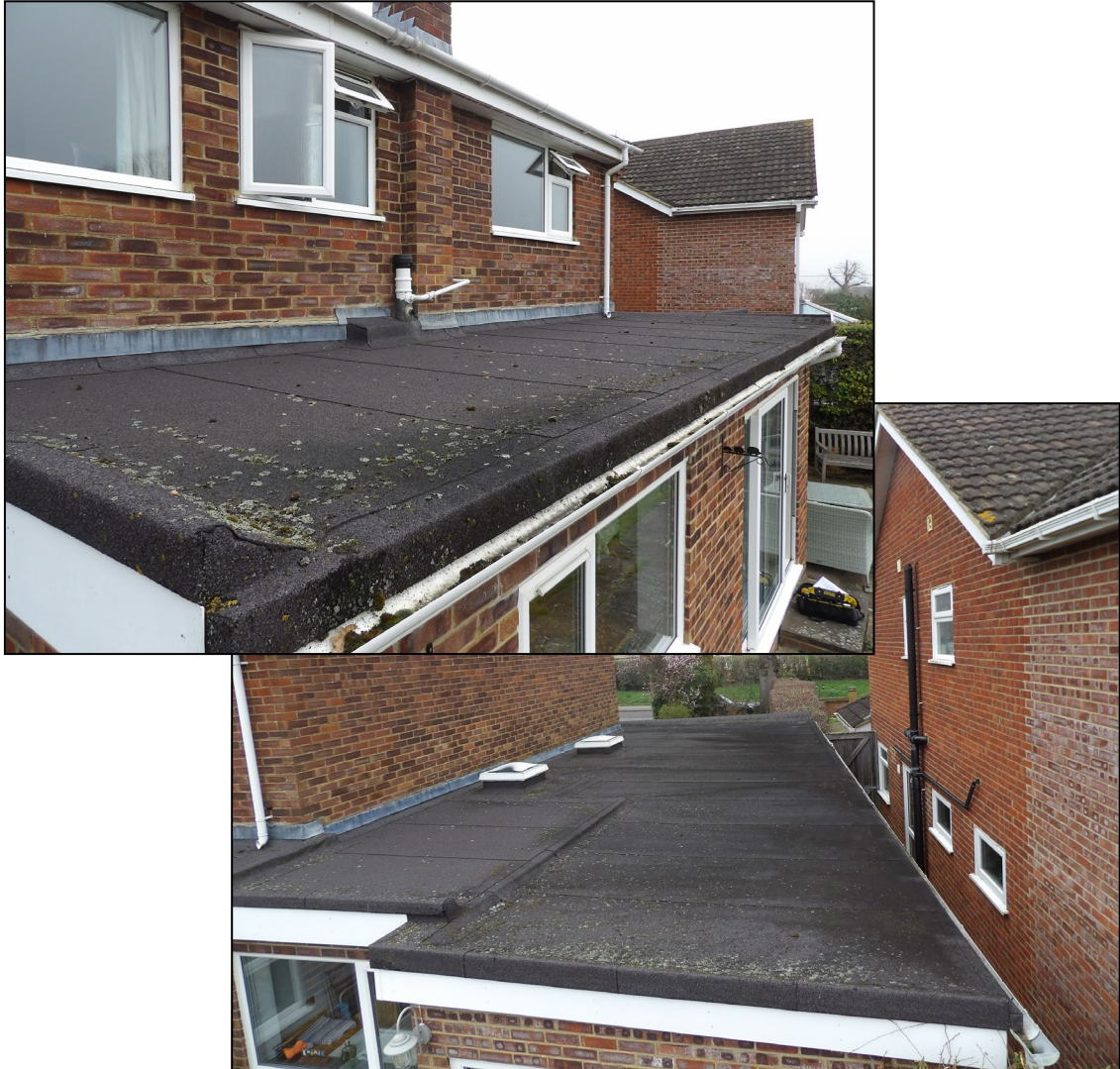
Figure 10. Example sealed uPVC soffits and fascias on single storey sections of the property. 44 Cutbush Lane, Shinfield. 04.03.26
