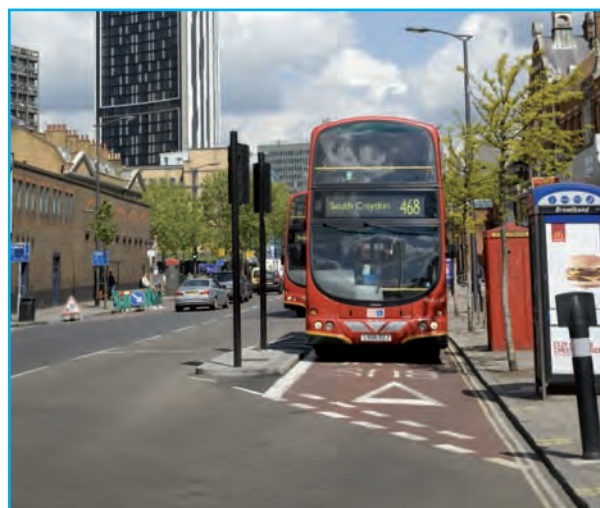
Bus Advance Area, Walworth Road MPR scheme
