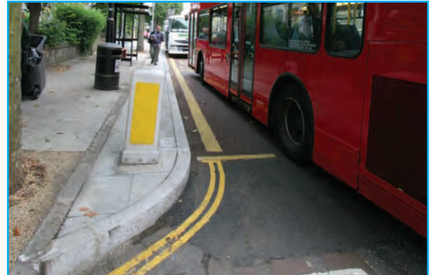
Reduced width bus boarder
