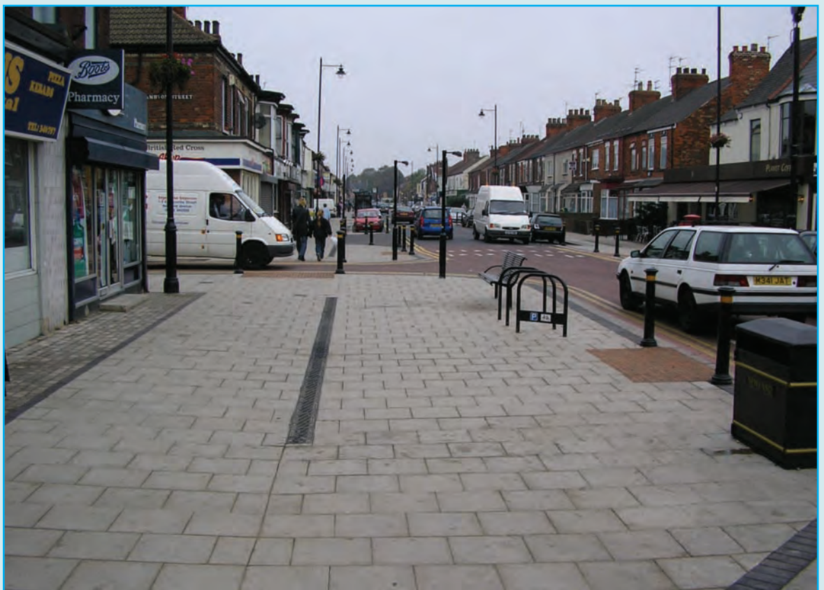
Footways widened significantly by narrowing carriageway
