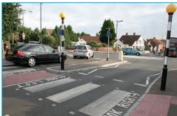
Zebra crossing close to mini-roundabout exit.
