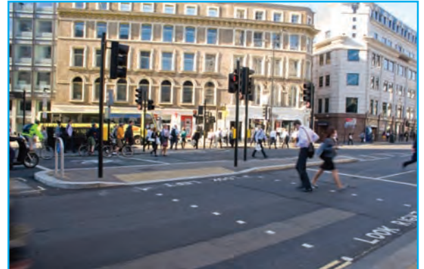
Staggered signalised crossing without guardrail
