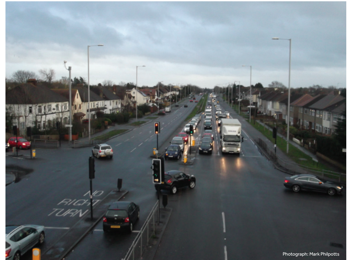
The A127 severs this suburban area
