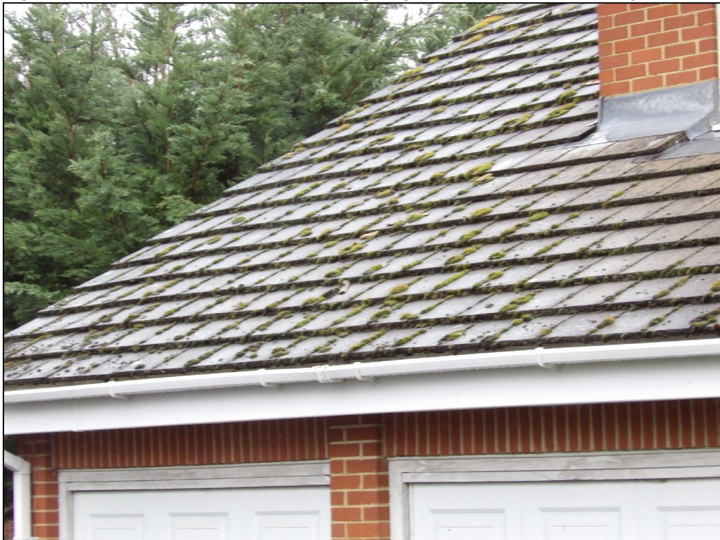
Figure 6. Example of roof tiles on porch/garage. 1 Beale Close, Wokingham. 15.01.26
