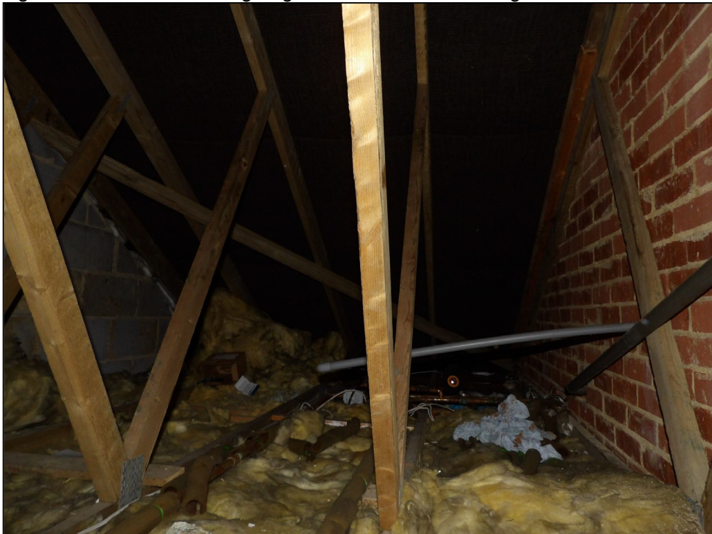
Figure 10. Loft void above garage. 1 Beale Close, Wokingham. 15.01.26
