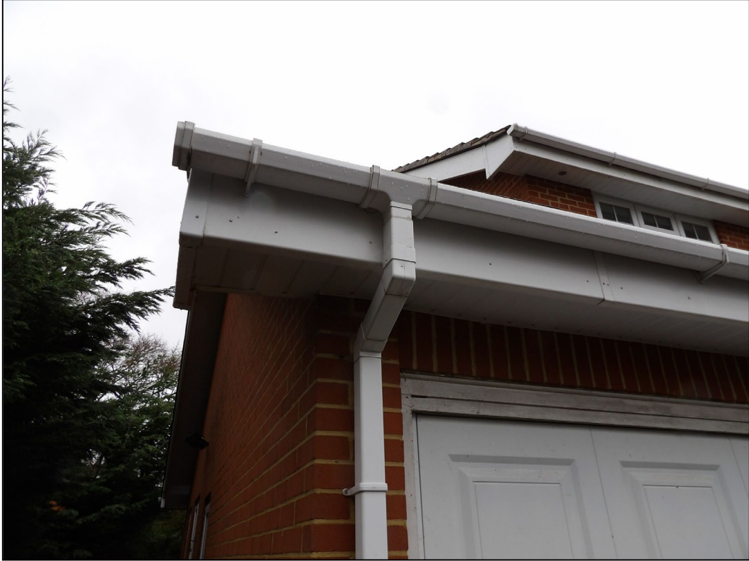
Figure 7. Example sealed uPVC soffits and fascias and cladding on property. 1 Beale Close, Wokingham. 15.01.26
