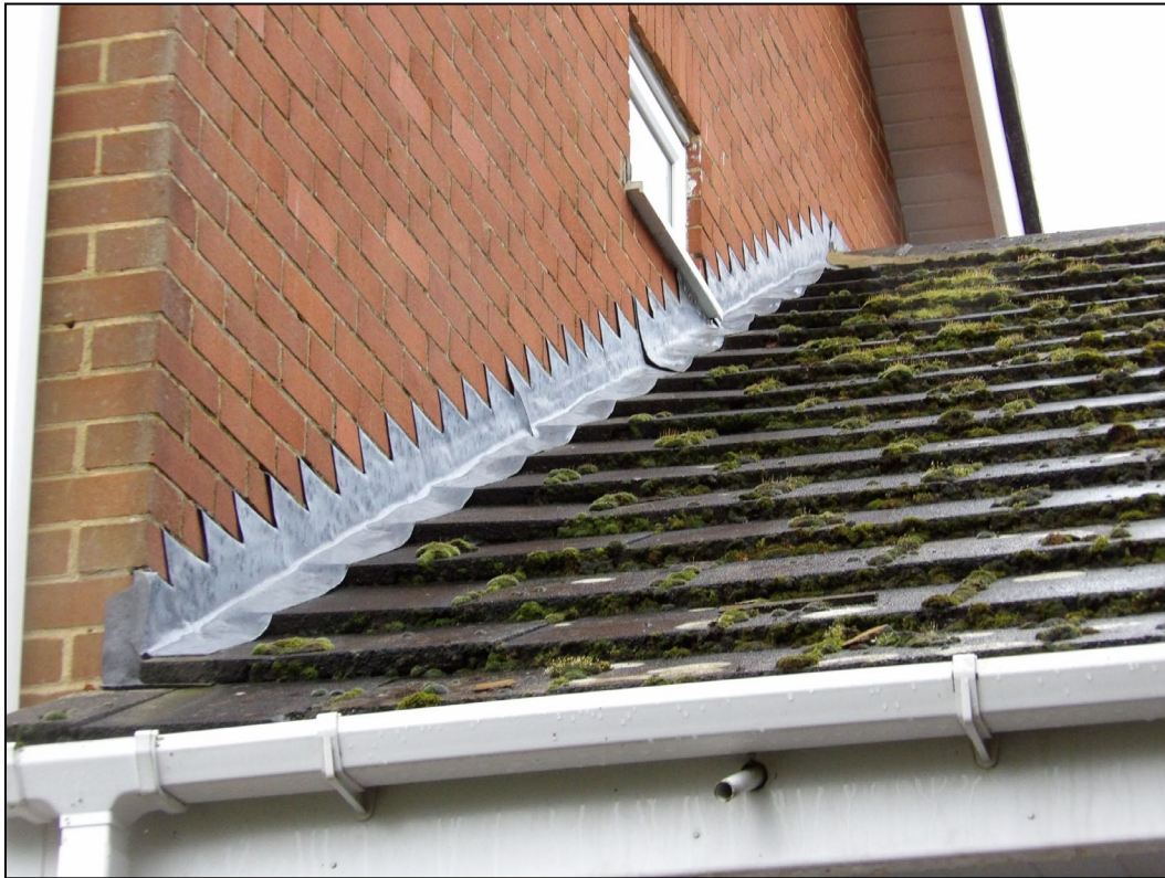
Figure 5. Example of sealed lead flashing. 1 Beale Close, Wokingham. 15.01.26
