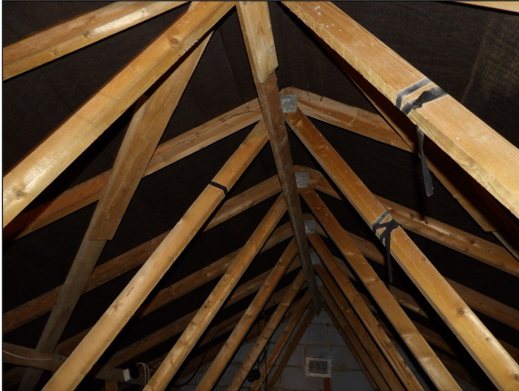
Figure 9. Example bitumen lining to main loft space. 1 Beale Close, Wokingham. 15.01.26
