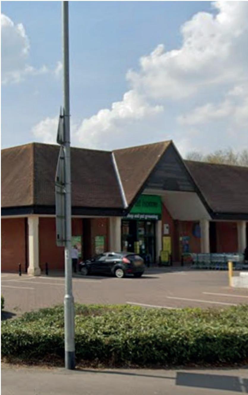
DEEP PROJECTING ROOF AT THE RETAIL PARK ON FINCHAMPSTEAD ROAD
