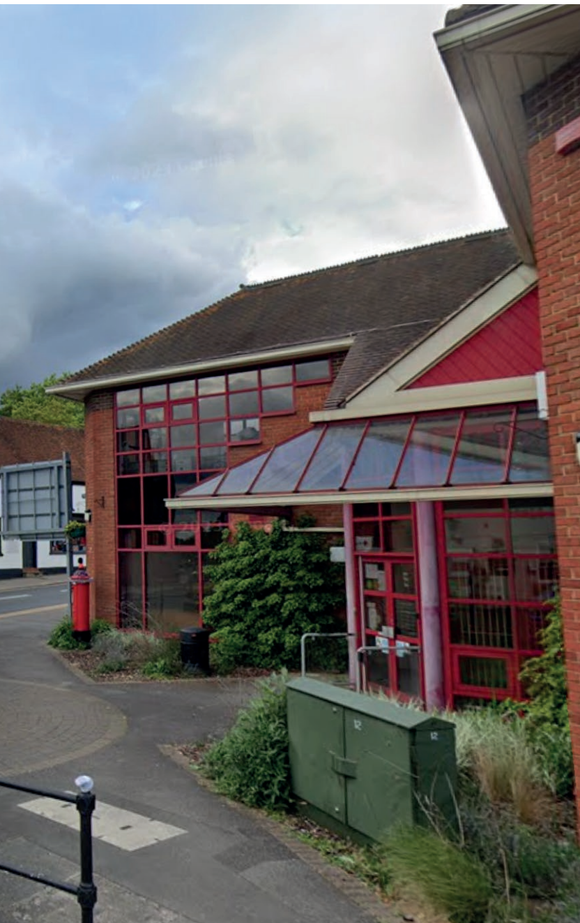
DEEP ROOF EAVES AT WOKINGHAM LIBRARY
