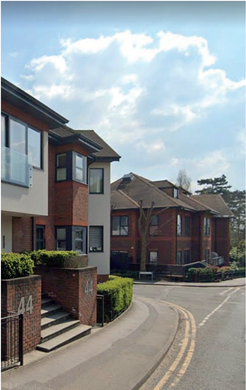
DEEP PROJECTING ROOF AT THE 44 FINCHAMPSTEAD ROAD
