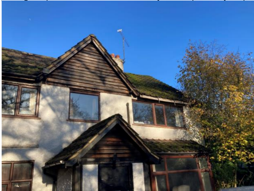
Photo 2 North east elevation
