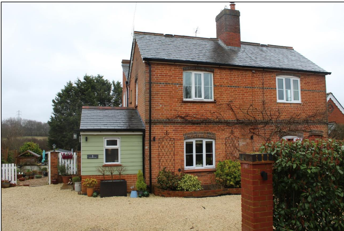
Photograph 1 – Front elevation as viewed from the front boundary
