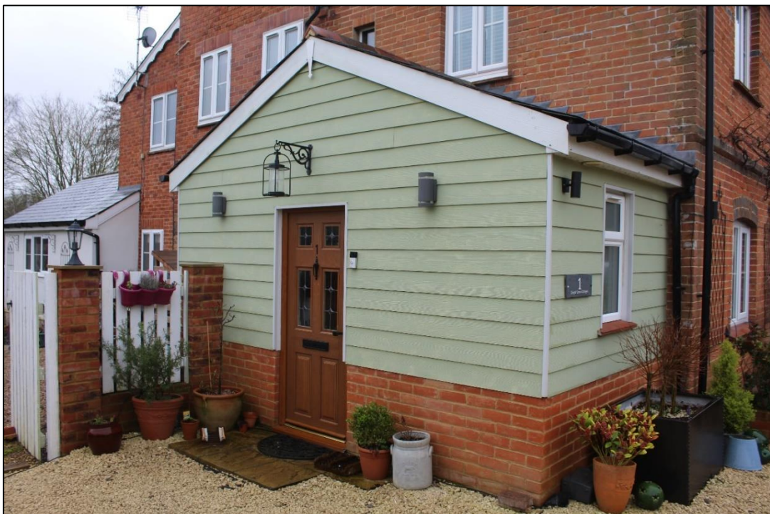
Photograph 3 – Front porch forming entrance and downstairs WC
