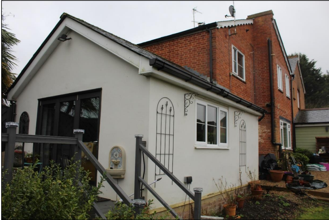
Photograph 2 – Single-storey rear extension forming sitting room
