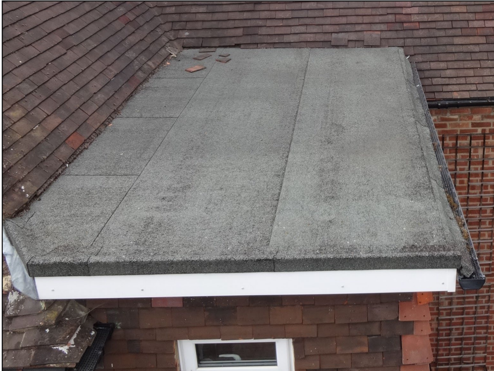
Figure 6. Bitumen covering flat roof extension. 3 Buckhurst Way, Earley. 26.08.25
