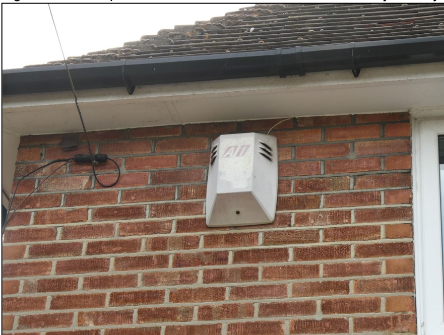
Figure 12. Example sealed soffits/fascias. 3 Buckhurst Way, Earley. 26.08.25
