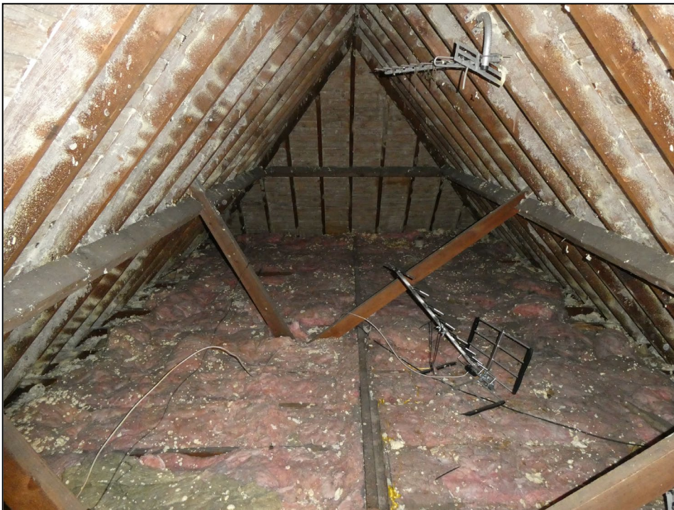
Figure 13. Loft space and sarking. 3 Buckhurst Way, Earley. 26.08.25
