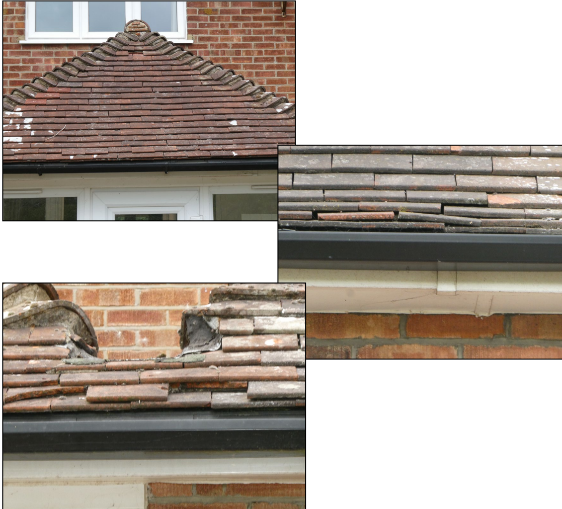
Figure 11. Example gaps in roof tiles on rear extensions. 3 Buckhurst Way, Earley. 26.08.25
