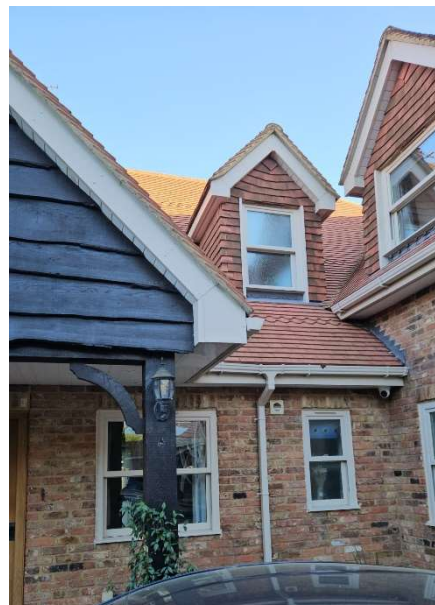
Photograph 2: North Elevation of CHH
