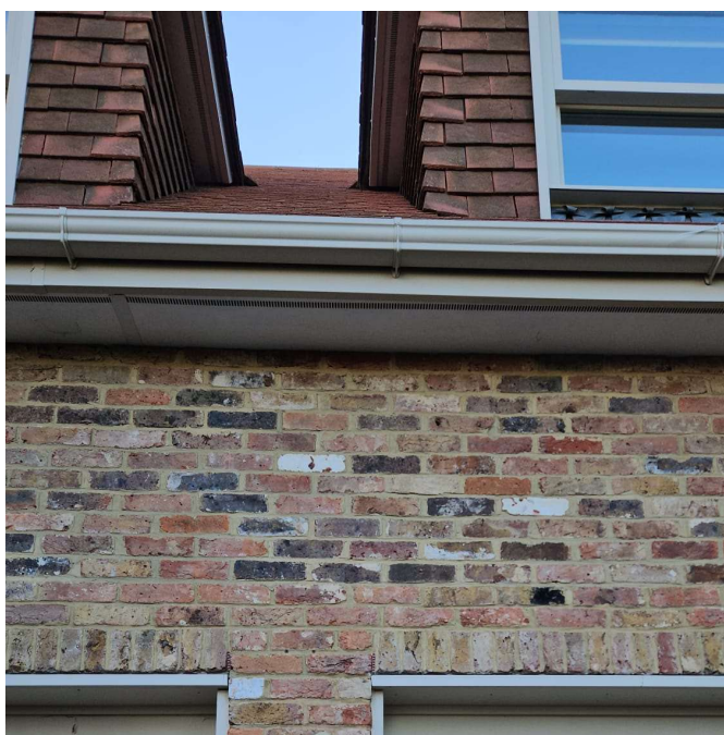
Photograph 14: External Eaves East Facing of CHH
