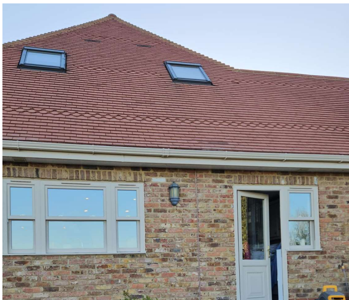
Photograph 15: External Eaves and roof tiles East Facing of CHH
