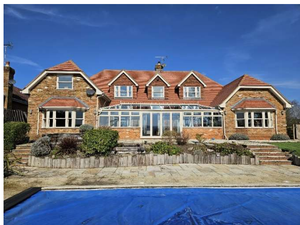
Photograph 3: South Elevation of CHH
