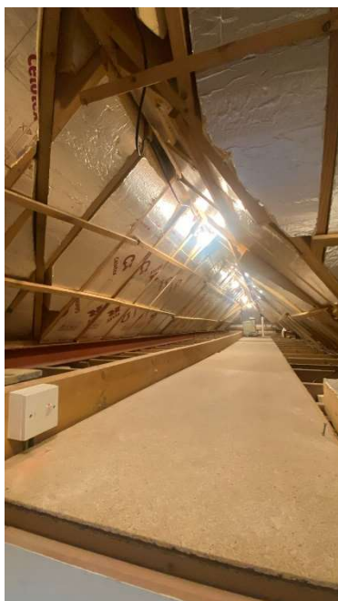
Photograph 7: Loft Void of CHH
