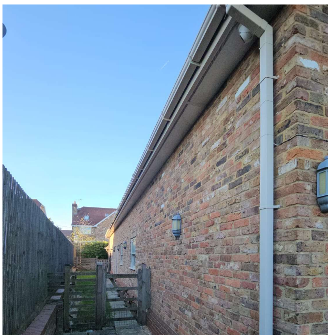
Photograph 13: External Eaves West Facing of CHH
