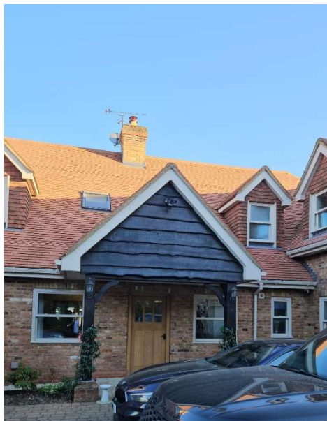
Photograph 1: North Elevation of CHH
