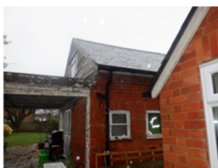
1. Front of the outbuilding from the south.
