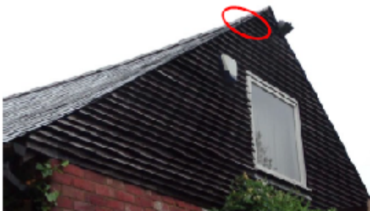
Photograph 1. Emergence location 1 (eastern gable)
