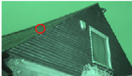
Photograph 2. Emergence location 2 (eastern gable)
