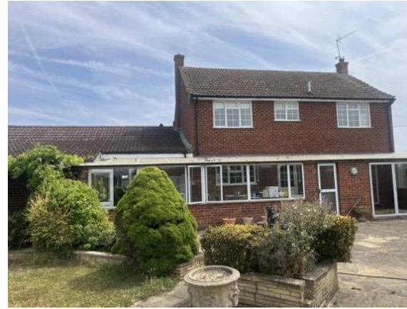
Building B1 - western elevation
