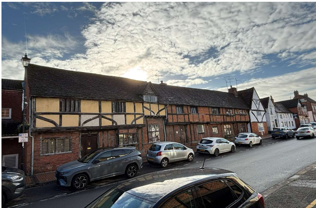
Figure 8: Front elevation of the Grade II* listed terrace of Nos. 33-39 (odd) Rose Street
