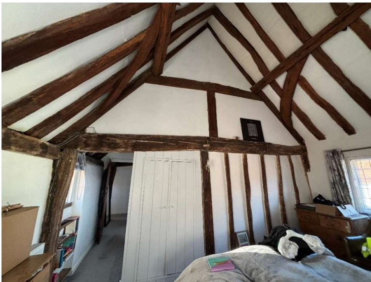
Figure 20: Framing in master bedroom; the insulation will reduce the depth of the timbers but they will remain clearly evident and a strong architectural feature.
