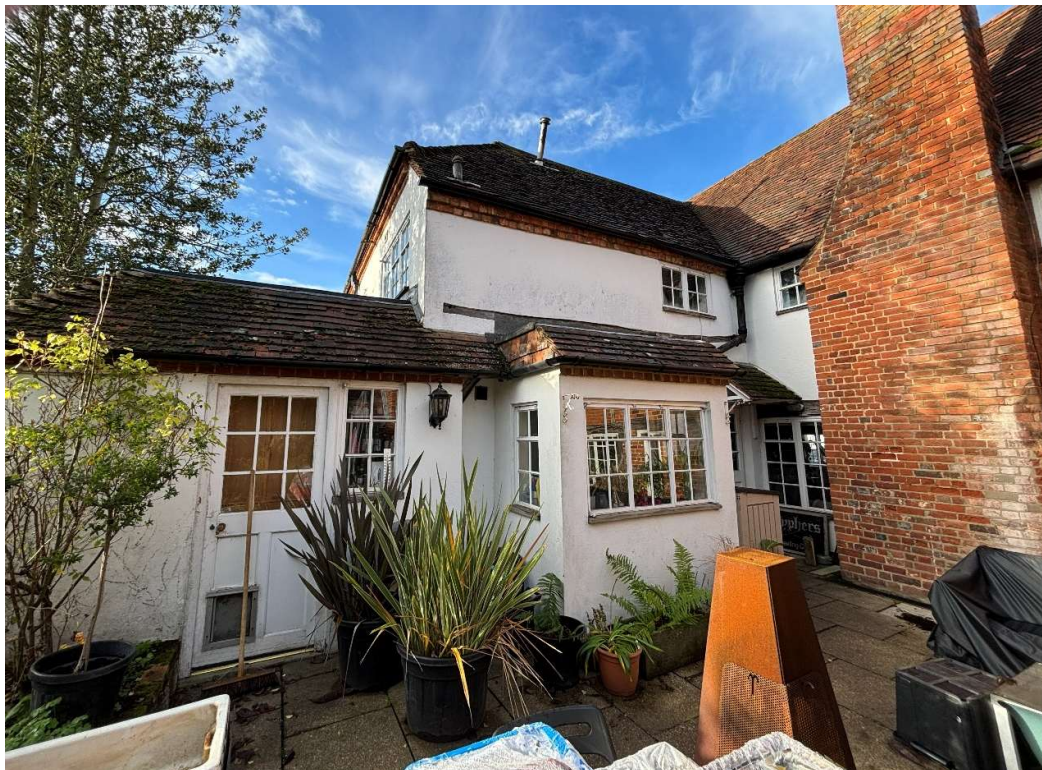
Figure 17 (top): Modern metal framed windows to the rear of historic range and Figure 18 (bottom): Matching metal casement windows in the modern extension
