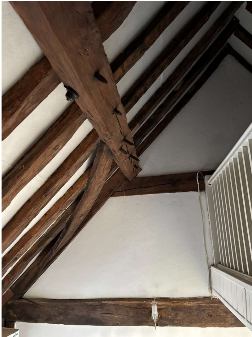
Figure 19: Timber framing at first floor; sitting proud of the modern hardboard panels used to enclose the roof structure, and create partitions between rooms
