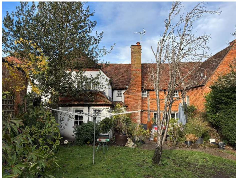
Figure 10: Rear elevation of No.37 Rose Street
