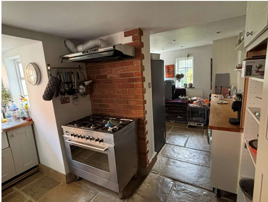
Figure 15: Internal view of modern extension showing wall nib to be removed
