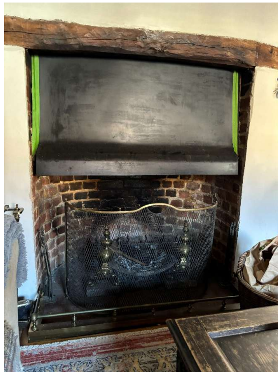
Figure 14: Fireplace showing brick hearth
