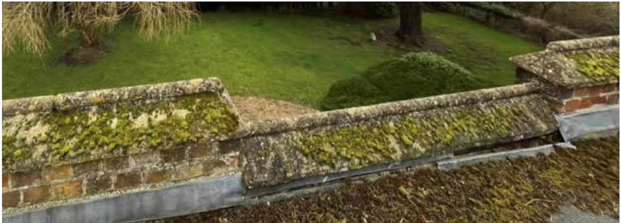
Front elevation – parapet with hipped ends to raised lengths of copings
