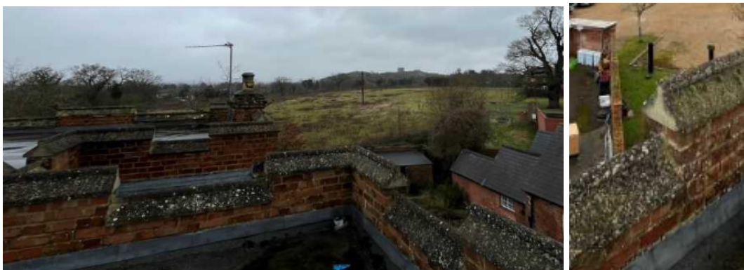
Rear elevation – raised copings have vertical ends to them except for corner returns. Rolled tops to coping
