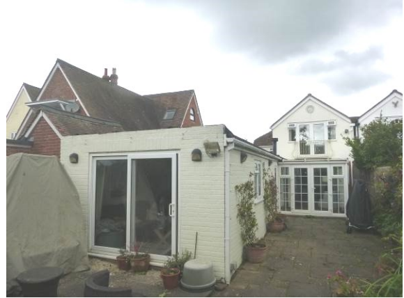
Photograph 2. Rear of property viewed from south.
