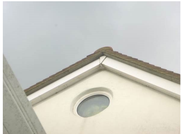
Photograph 4. Tight uPVC barge boards on rear gable end (rear elevation).
