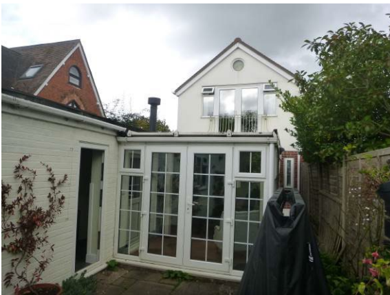
Photograph 5. Rear conservatory (rear elevation).
