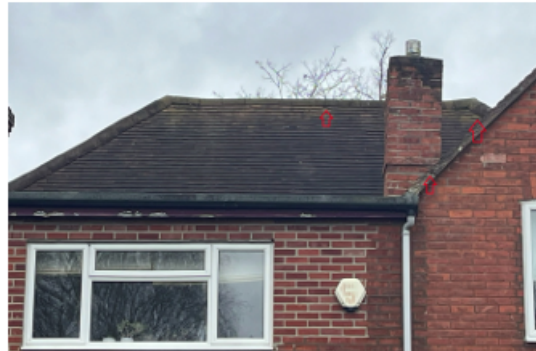
Figure 6. Southern elevations looking north: red arrows indicate potential openings which bats could exploit
