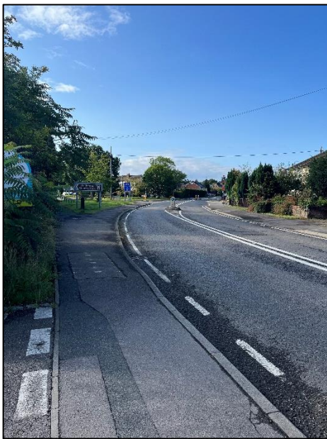
Photograph 1: Existing conditions along Basingstoke Road/B3349
