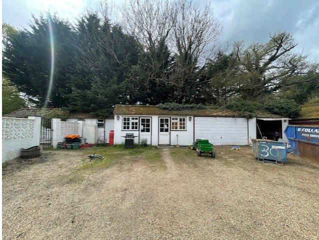
Photo 6 – View of front elevation of outbuilding (northeast)
