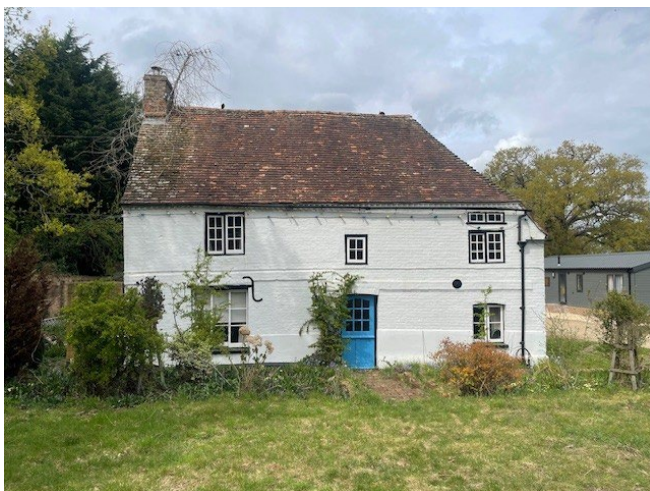
Photo 5 – View of side elevation (southeast)
