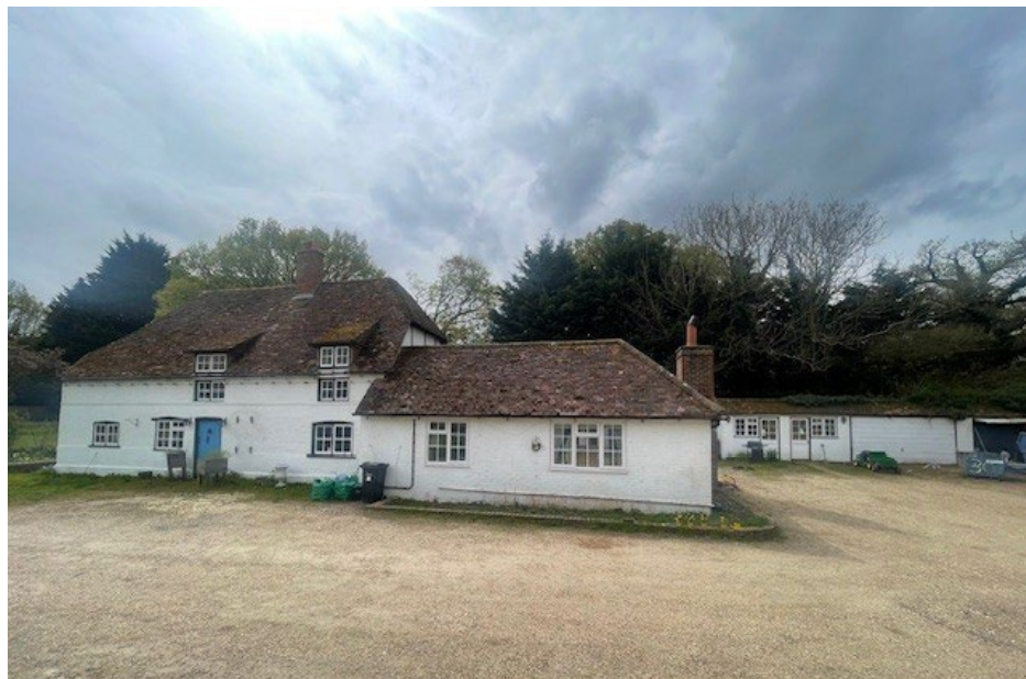
Photo 1 – View of front elevation (northeast)
