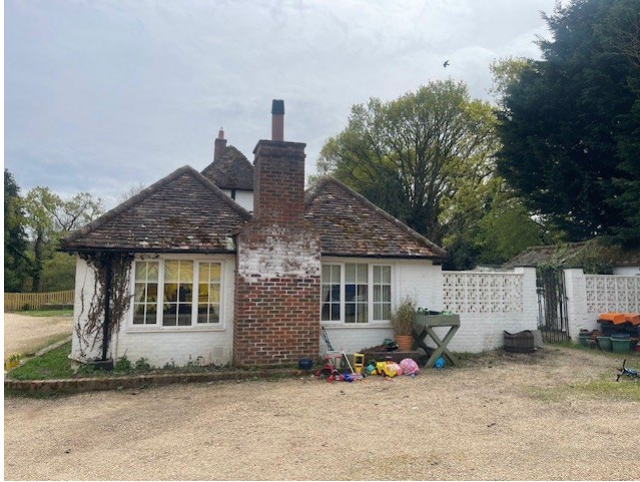
Photo 2 – View of side elevation (northwest)
