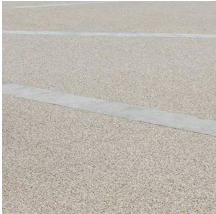
Light-coloured buff bonded gravel provides a robust surface suitable for vehicles
