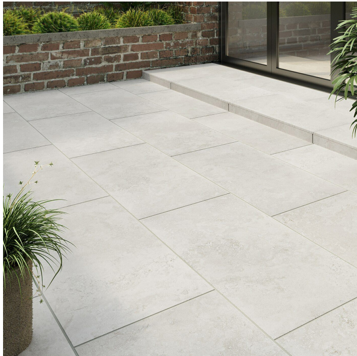
Light grey porcelain paving to the external pedestrian areas
