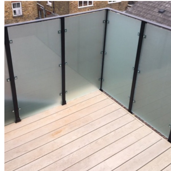
Terrace privacy screens formed of obscured glazing
