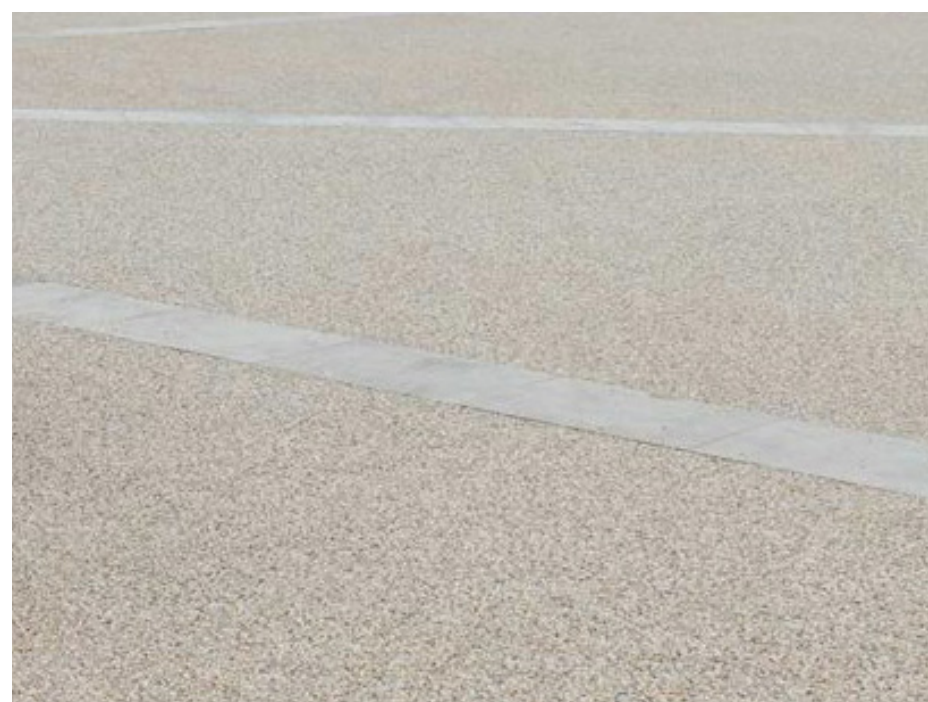
Light-coloured buff bonded gravel provides a robust surface suitable for vehicles
